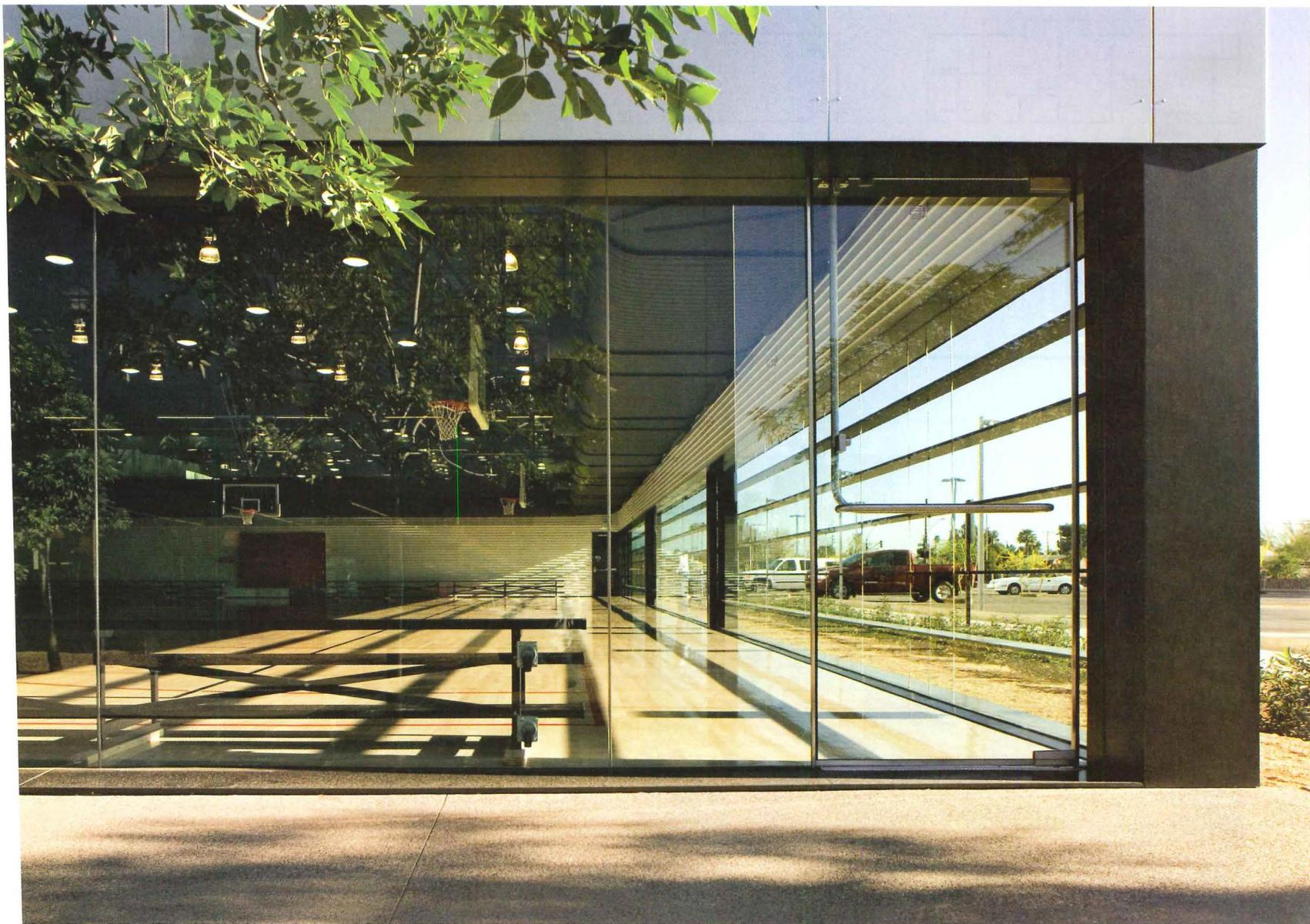
**Horizontal louvers shade glazing on the gym's east side (above). The breezeway turns into a corridor inside the building (right).**
