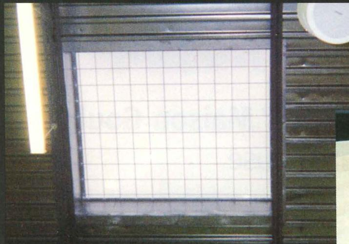
OSHA approved! Interior Safety Screen mounting, instead of exterior mounting, eliminates additional jobsite labor because the screen is built into the RPI structural curb. Saves cost, provides clean exterior look, and offers maximum security against entry. Curb can be manufactured to any bar joist spacing, which eliminates reinforcing. RPI can also supply the skylights, or, just the screens to be mounted inside existing curbs.
