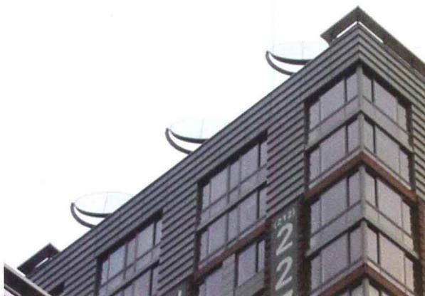
At Battery Park City's Teardrop Park, Carpenter Norris Consulting installed three heliostats (left and below two) to bring daylight into a secluded urban landscape. The mirrors track the sun and reflect elliptical-shaped spots of daylight—at nearly 90 percent of the sun's brightness—onto eighteen places in the park. Alternately, fiber-optic cable (bottom) is used by Parans to bring daylight to otherwise conventional-looking light fixtures deep within a building.
