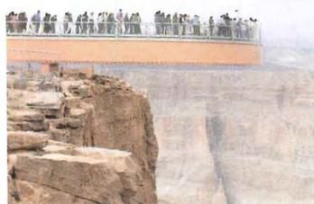
The viewing platform projects over a relatively narrow side canyon known as Eagle Point. Two large box beams, composed of 21 welded pieces, form the horseshoe-shaped structure; steel caissons, attached to piles drilled 40 feet into thick limestone, anchor them. Johnson says its shape was developed to maximize visitors' perception of the dramatic surroundings—and the sensation that they are floating over the canyon.
