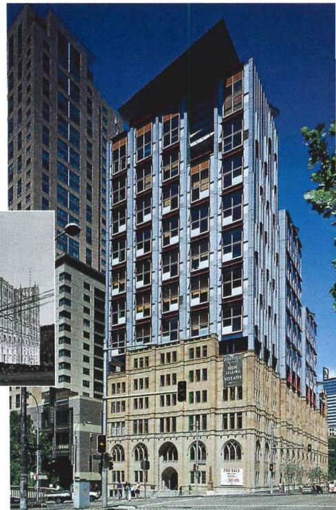
walls made of plaster instead of masonry (due to the load constraints), the 1926 base could support the weight of the new structure and its occupants.
