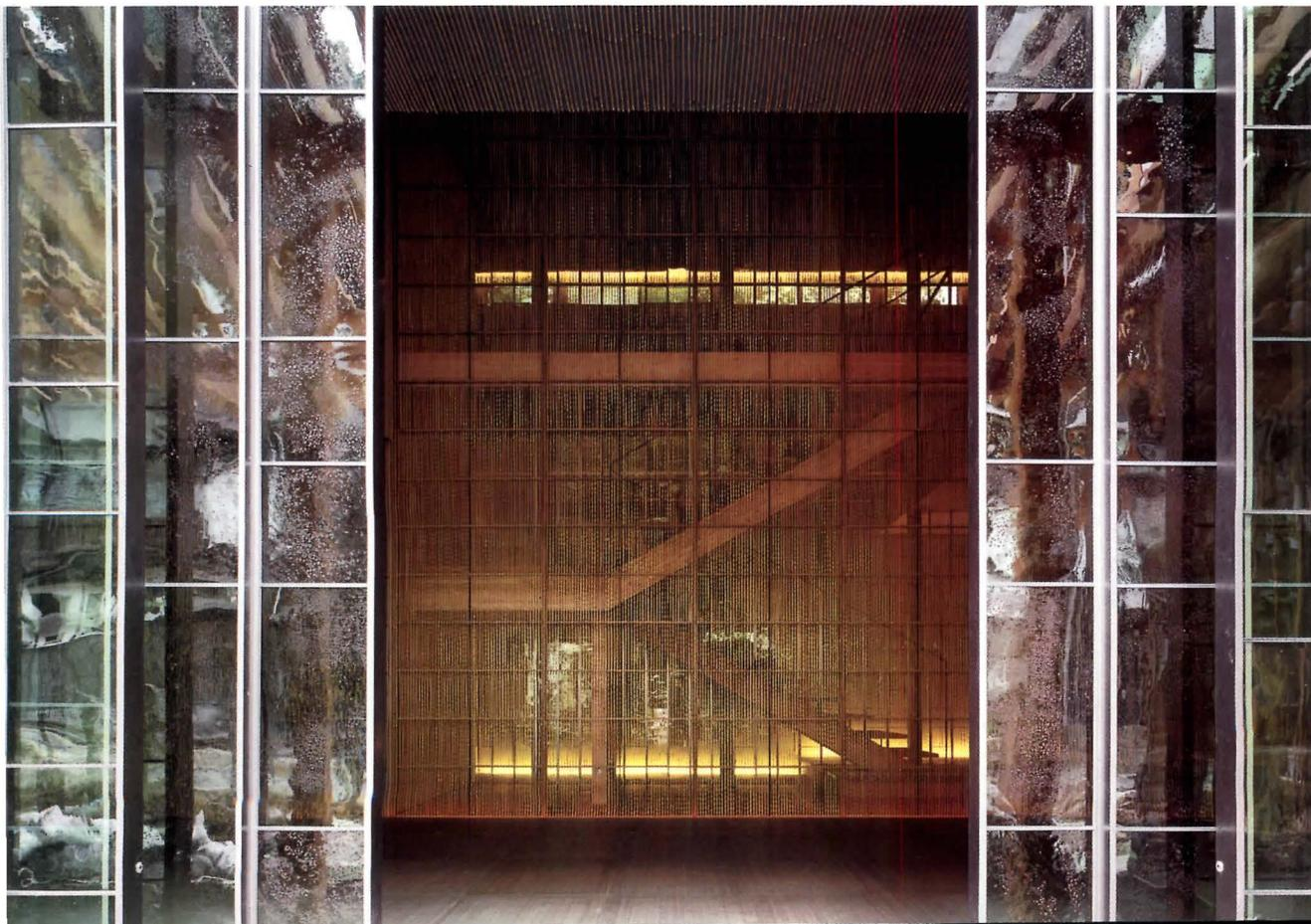
Subtly lit treads suspended from the ceiling on steel rods give a stair connecting the top two floors a sense of floating in space (above). A 700-year-old French handblowing technique called *dalle de verre* was used to create part of the almost-transparent glass entry wall (left).
