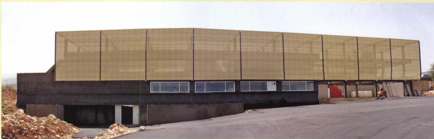
In the village of Kfifane, Sarkis designed an olive-oil-press building whose external veil prevents direct light from hitting the press equipment. Inside, a viewing platform allows farmers to follow the oil-pressing process.
