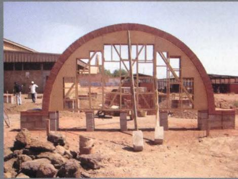
Vegetable vendors occupy many of the market's stalls (above). Compressed earth blocks, formed with a hand-press machine, were used for roofs as well as for walls (far left). Large arches support dome-shaped roofs (left).
