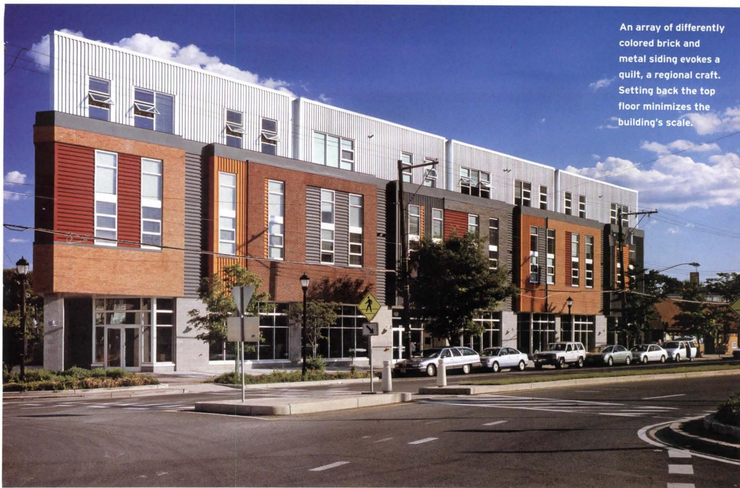
An array of differently colored brick and metal siding evokes a quilt, a regional craft. Setting back the top floor minimizes the building's scale.
