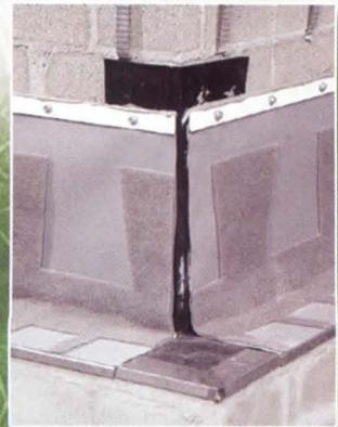
Uses 40-mil polymeric, reinforced, UV stable flashing membrane, incorporating DuPont's Elvaloy® KEE polymer.
