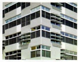
NBBJ occupies the first three floors of the office building (top and opposite, top). Automated sunscreens (left) and reflector blinds (above) alternately slow heat gain and allow daylighting.
