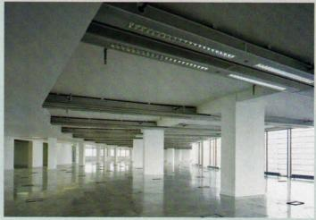
A sciences building designed by Zimmer Gunsul Frasca for the California Polytechnic State University (above left) will have naturally ventilated offices and laboratories heated and cooled with active chilled heams. For the conversion of a hotel into the **Empress State office building** (right and above), in London, Wilkinson Eyre Architects chose multiservice chilled beams (left), which combine cooling, lighting, and sprinklers, among other features, in an integrated enclosure.
