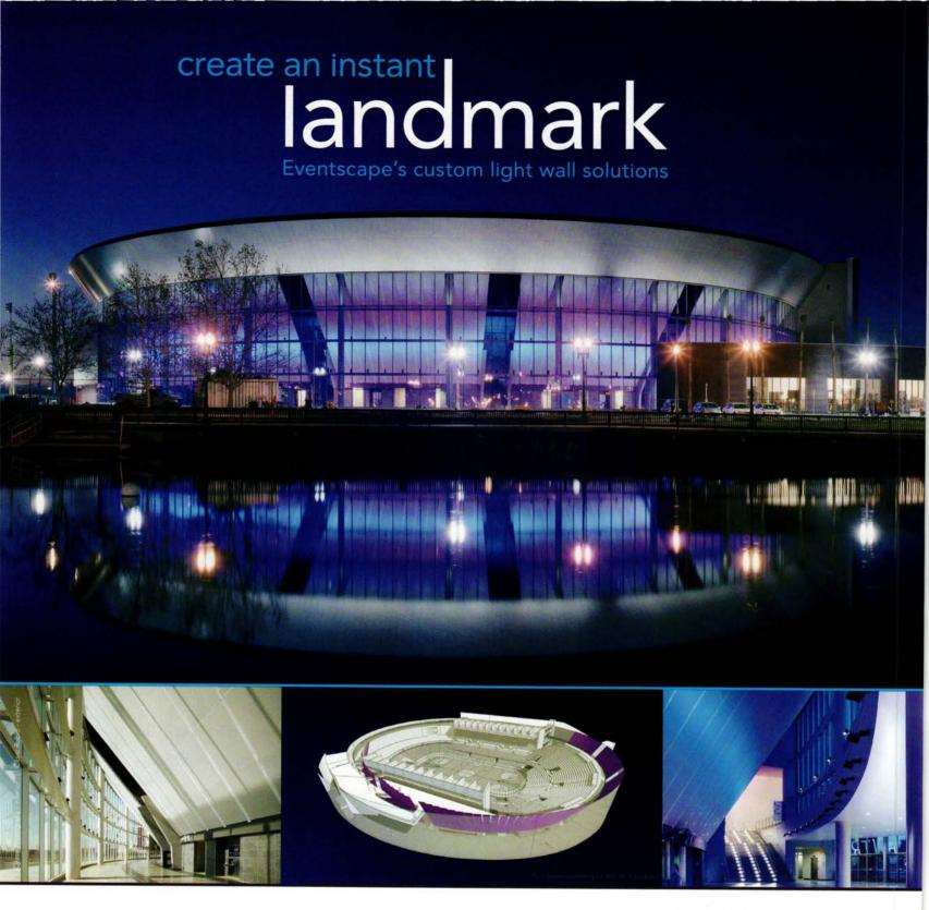
Stockton Event Center - CA | Custom sloping wall - panelized frame & coated fiberglass fabric | 45'H x 480'W - 21,000 sq. ft. | Eventscape - fabrication | 360 Architecture - design
