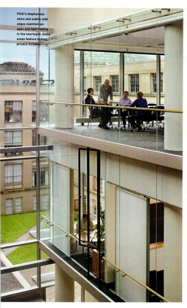
views and improved circulation for adjacent spaces. Wrapped on all sides in glass, including extensive skylights, the building's diaphanous facades are articulated by brisesoleils, operable windows, and translucent sliding screens. Metal baffles in the ceilings further that open feeling. PDSI is one of the first American buildings to incorporate highly efficient chilled beams, which are visible just above the baffles (see technology article, page 182).
