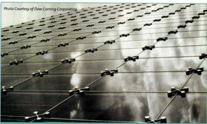
The world's first four-sided silicone structural glazing project. The metal ornamentation is for decorative purposes only, and does not provide structural support.
