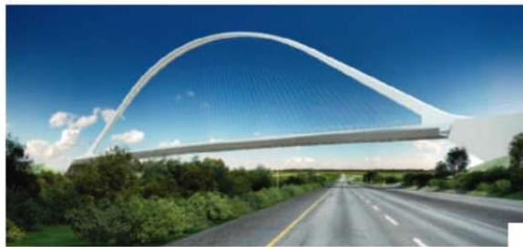
deck hangs from a single arch by cables and supports flanking orthotropic decks on steel ribs. According to engineer Gabriel Calatrava, Santiago Calatrava's son, the bridge's deck – without train tracks – will most likely be manufactured off-site and then "launched" into place, using temporary supports to limit traffic disruptions on Peña Boulevard.
