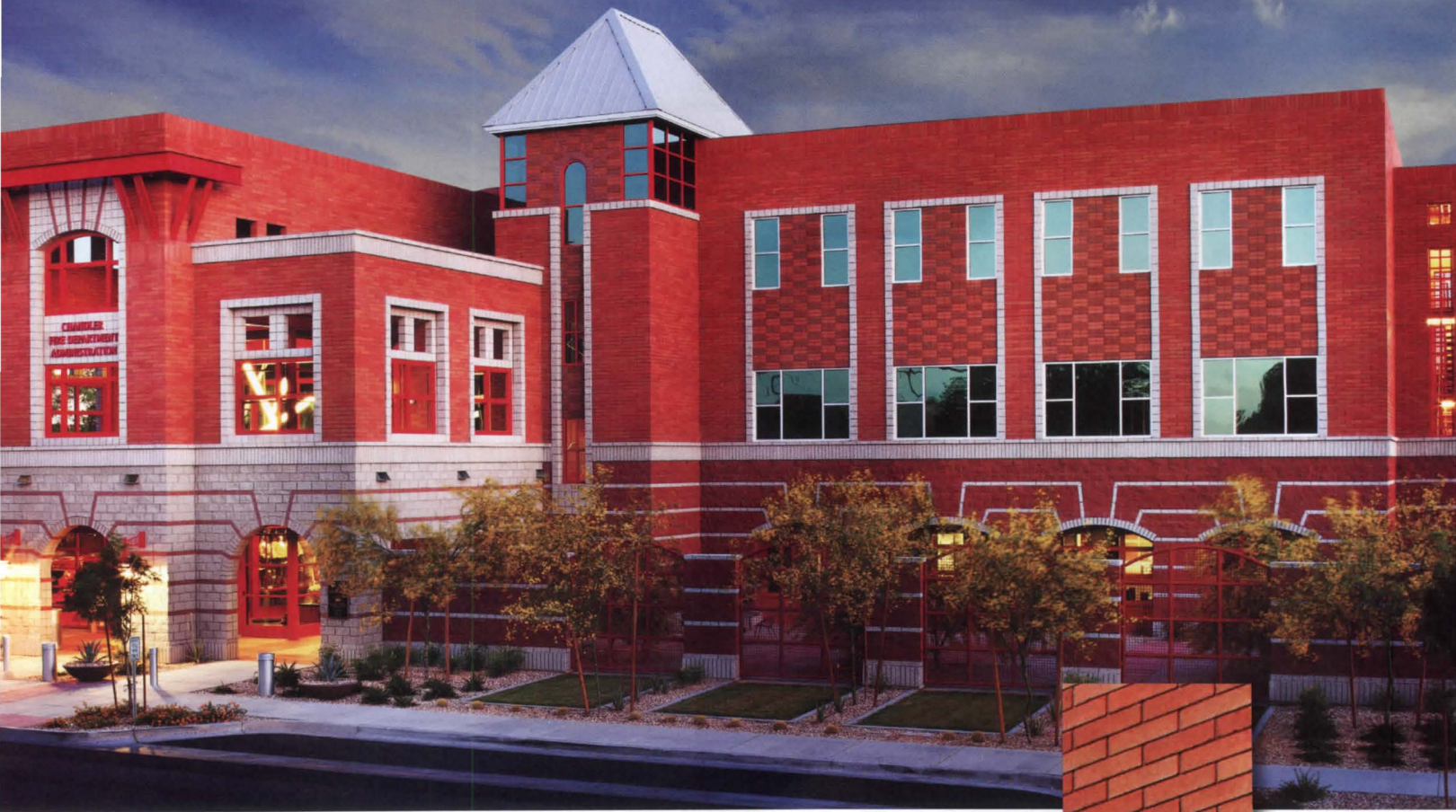
-Project: Chandler Fire Administration Building, Chandler, AZ.
