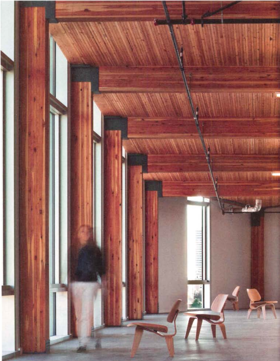
LOFTLIKE The 14-foot floor-to-floor dimension, full-height windows, and exposed heavy-timber structural components give the Bullitt's interior spaces an open and decidedly regional quality.
