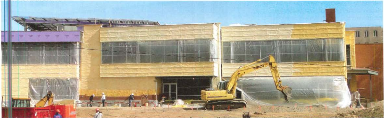
Medium-density closed cell insulation can be spray applied to the outside of the sheathing on a stud cavity wall assembly and remain durable and water resistant during the construction period.
