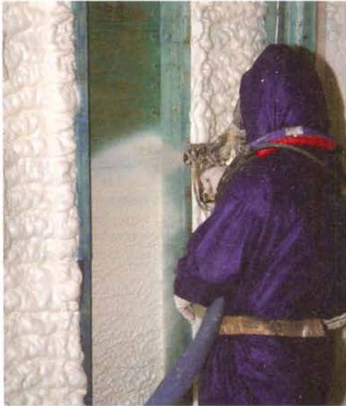
Spray foam insulation is mixed on site and applied using spray gun equipment appropriate to a particular manufacturer.
