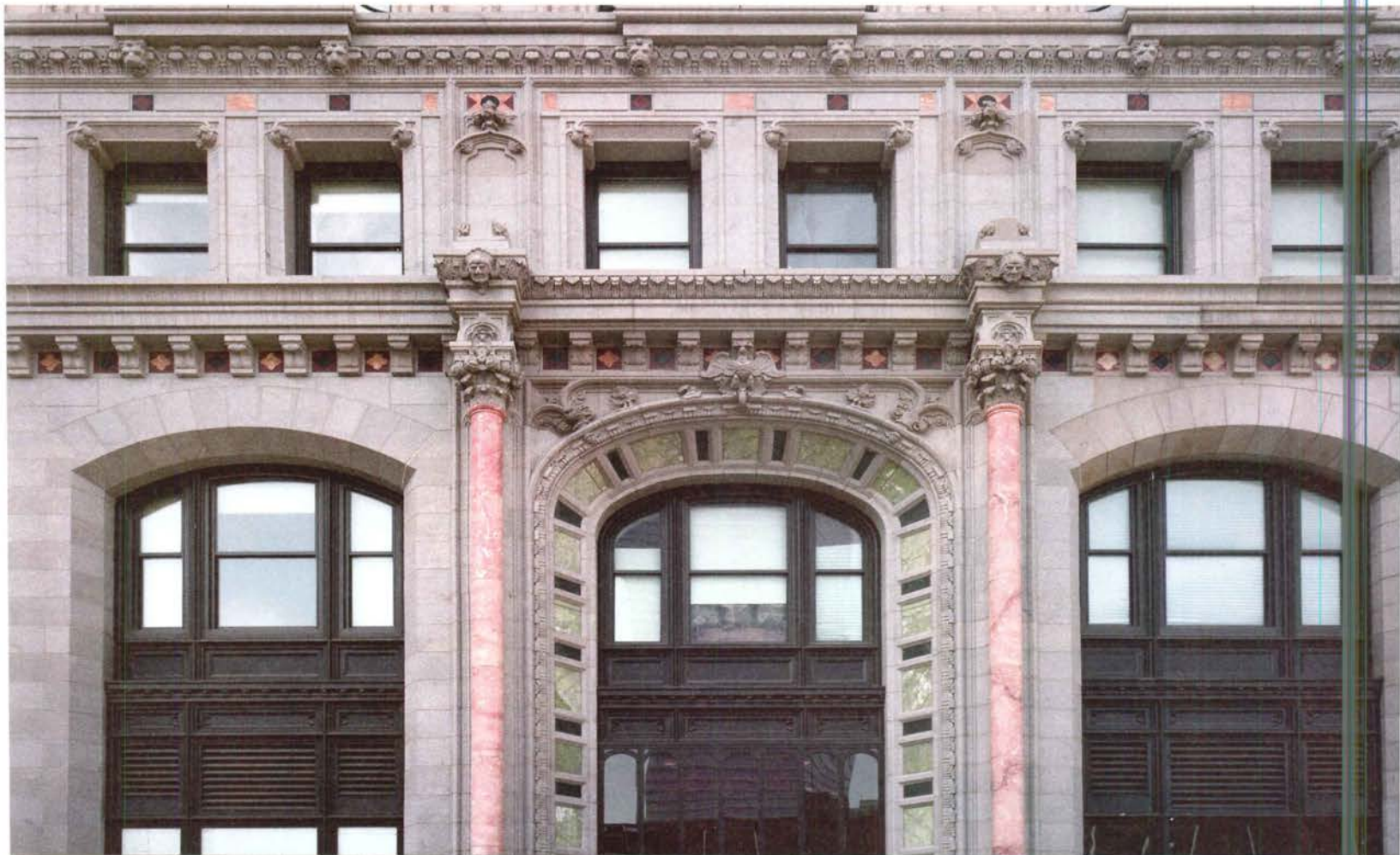
90 WEST STREET RENOVATION - NEW YORK CITY, NY
