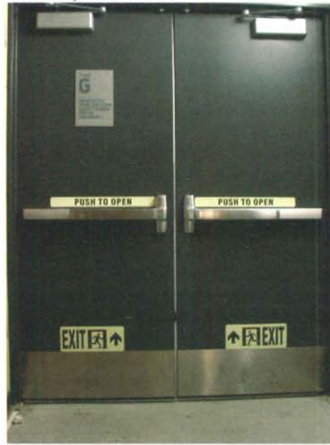
New York City's Barclays Center emergency stairwell exit door with markings
