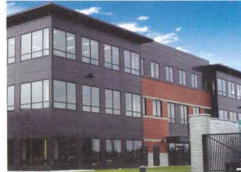
As a government project, the Fort Knox Human Resource Center had to work within a limited budget and meet a minimum LEED Silver design certification.
