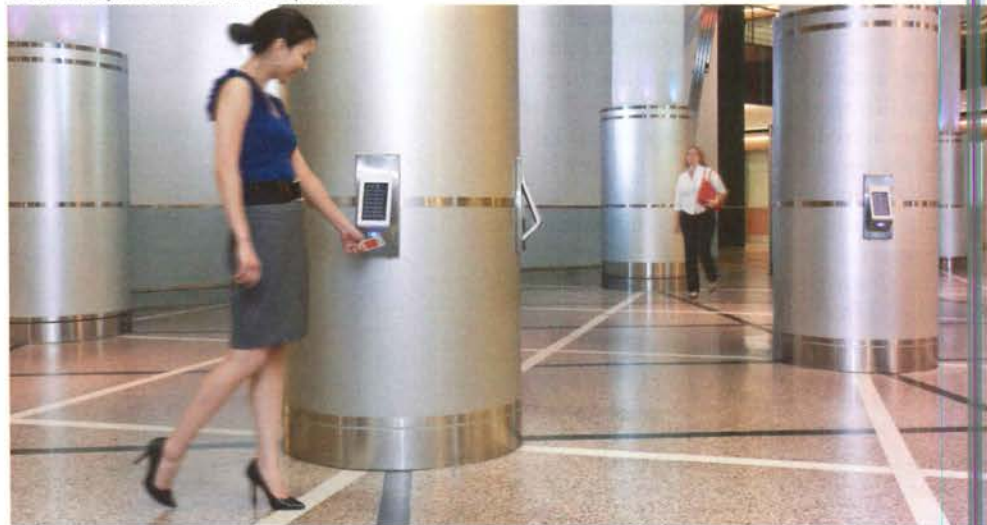
The addition of access-card readers to the user control panel allows customized service.
