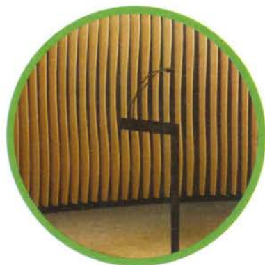
Sculptural wall fins fabricated from wood elements create an undulating 3D form while dispersing sound waves to enhance acoustic performance in the circular Bechtel Conference Center at the Public Policy Institute of California.
