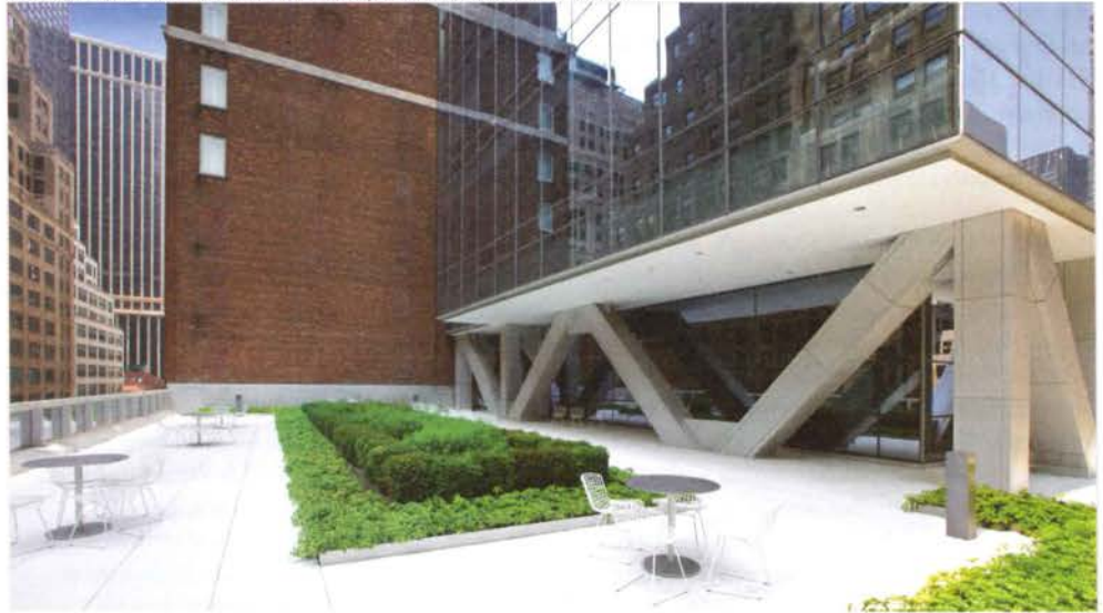
The story-tall transfer girders above the fifth floor help create a roof garden at 510 Madison Ave.
