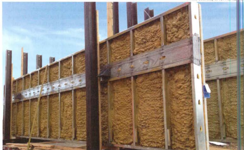
Low-density open cell spray foam insulation has been installed to fill and seal stud cavities of this prefabricated wall panel and shipped to the site for final installation.
