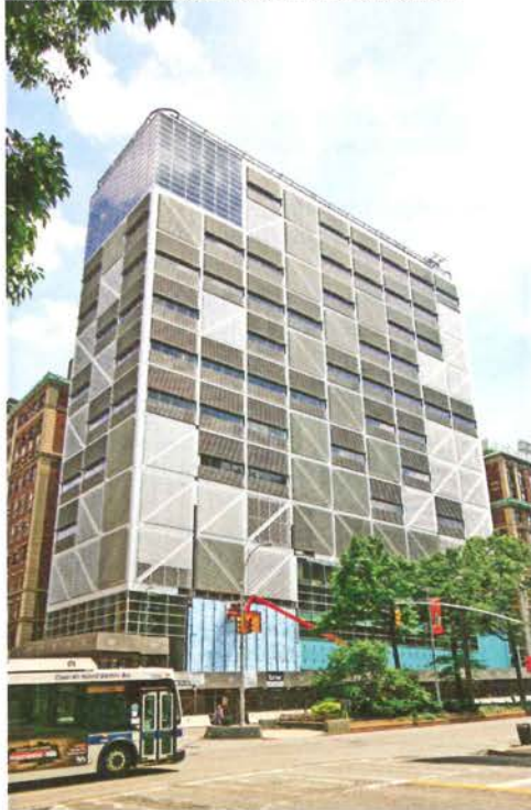
The Northwest Corner Building at Columbia University in New York City needed to span over an existing gymnasium to create the needed space in the upper floors.
