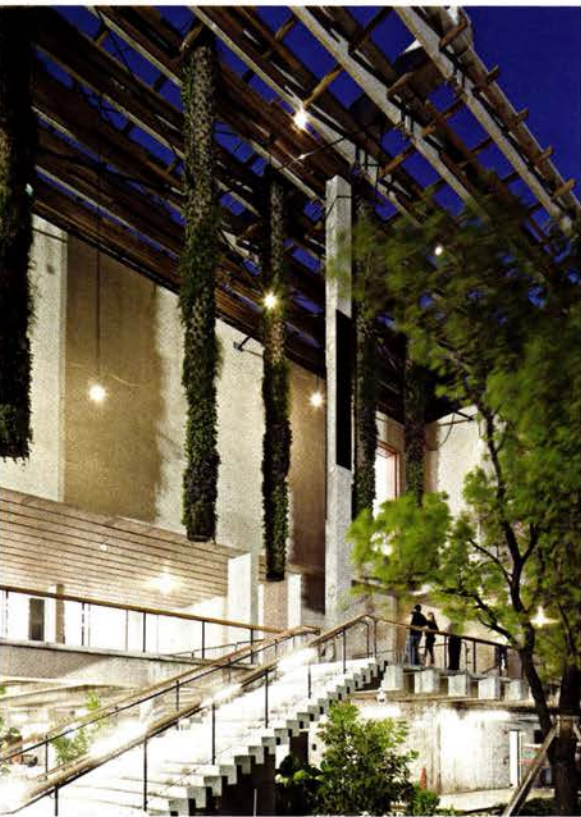
Thin concrete columns support a wood canopy hung with strands of vegetation.
