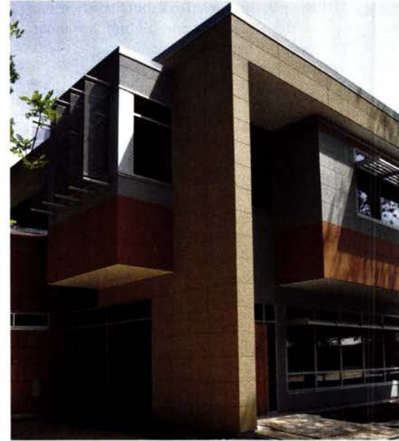
Bold colors were used on a new facility for St. Francis High School in Wheaton, Illinois, designed by Serena Sturm Architects of Chicago and the architect-academic Keelan Kaiser, AIA, using cement-fiber panels in a high-performance envelope.
