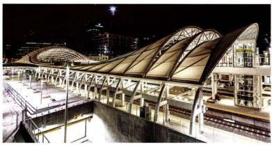
Ventilation towers for the underground bus station are located next to the light-rail platform (left). A 500-foot-long fabric canopy shades the train platform (right).
