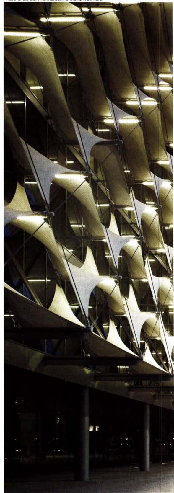
In Riyadh, Saudi Arabia, a glass-enclosed expansion to the King Fahd National Library was complemented by a woven glass-fiber membrane made of 1,000 twisted square awnings that block 93 percent of the incoming sunlight.
