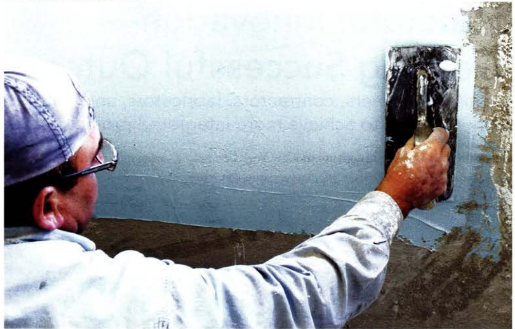
Fluid-applied membrane systems can be applied to an appropriate substrate by using a trowel, a roller, or a sprayer as field conditions may warrant.
