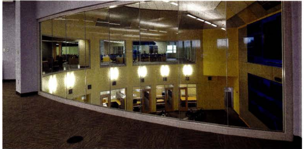
Laminated safety glass, fire-protective glass, and fire-resistive glass all allow light and views to pass through from space to space while meeting a range of fire code and security requirements.
