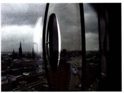
America, which engineers and installs complex facade systems. The process of heating the glass, draping it over a mold, then cooling it down, demands enormous attention to maintaining exact dimensions and avoiding surface distortion.
