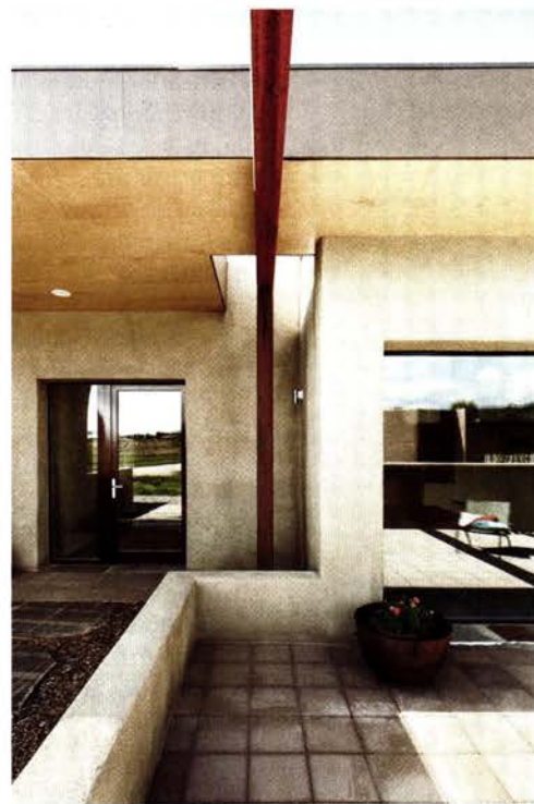
TAOS HOUSE This desert house (top and above) has overhangs that protect it from unwanted heat gain. Architects from NEEDBASED supported the projecting elements with steel portal structures that do not penetrate the envelope, helping prevent thermal bridging.
