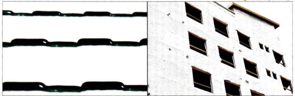
Strategically located spacers provide an intended drainage gap on synthetic, non-woven, breathable water-resistive barriers.
