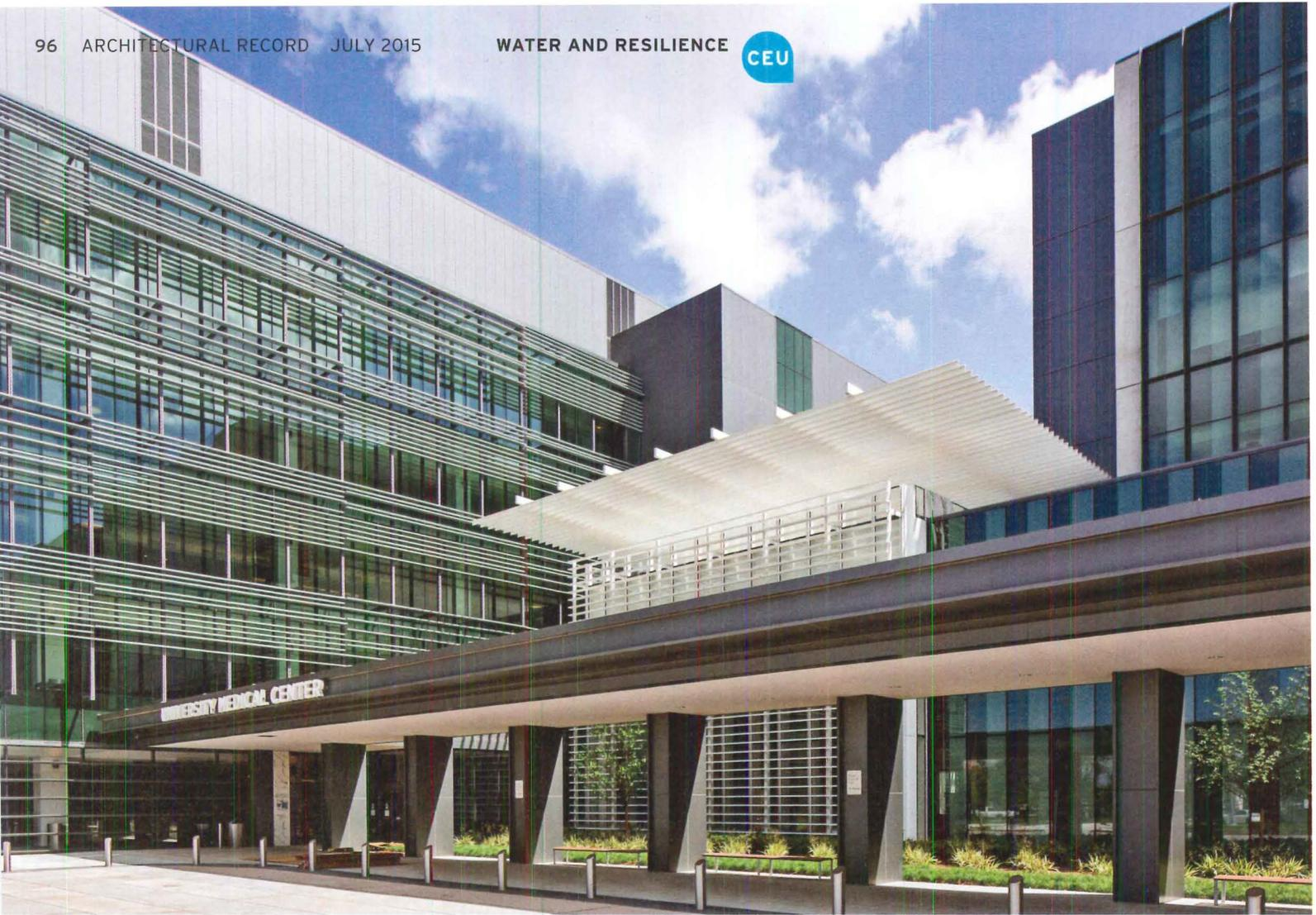
**MISSION CRITICAL** At University Medical Center (above), the NBBJ-led design team placed no critical functions or essential mechanical systems on the ground floor. Eskew+Dumez+Ripple designed an emergency suite above flood level at New Orleans East Hospital (below). A vehicle access ramp can double as a boat launch if needed.
