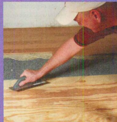
up to ¼ inch from concrete subfloors to the covered flooring material. It also includes an antimicrobial additive that inhibits mold growth and, with an R-value of approximately 0.50, adds a bit of a thermal break to the flooring assembly.
