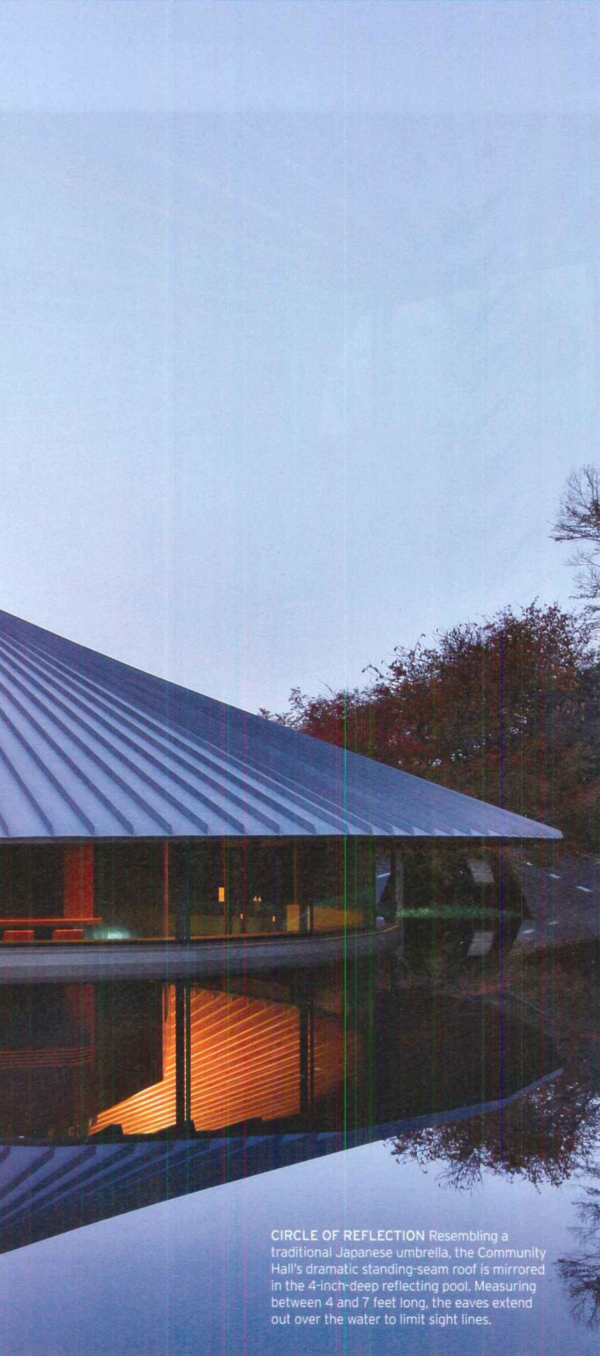
**CIRCLE OF REFLECTION** Resembling a traditional Japanese umbrella, the Community Hall's dramatic standing-seam roof is mirrored in the 4-inch-deep reflecting pool. Measuring between 4 and 7 feet long, the eaves extend out over the water to limit sight lines.
