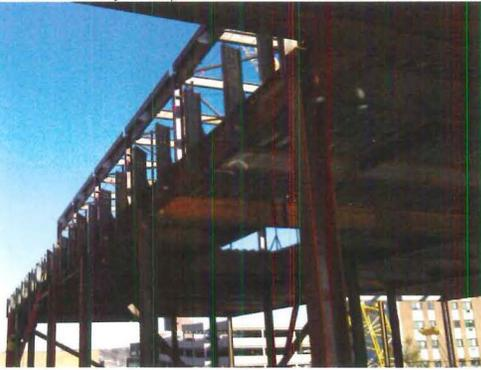
At the State University of New York Institute of Human Performance Upstate Medical University, structural steel was selected for this laboratory expansion project. Pictured above, upper floor and mechanical penthouse levels of the steel frame with horizontal bracing members at the roof and attachments will support a tied-back infill skylight. In the photo to the right, the full-story transfer girders serving as an interstitial-level MEP services distribution zone can be seen.
