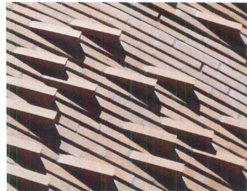
dry-pressed bricks, a variation on molded bricks, which enabled the intricate shapes to be formed.
