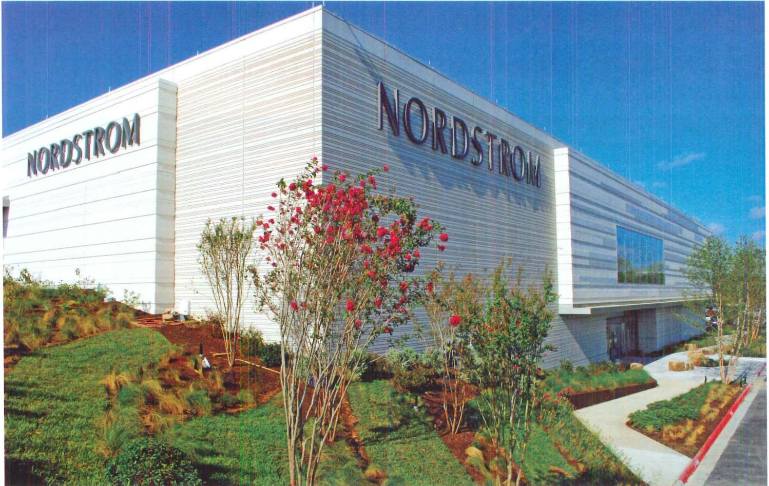
Nordstrom is using precast concrete to create its new high-performance enclosure system that is being used in all of the stores around the country. The precast panels provide edge-to-edge, continuous insulation and serve as the air and vapor barrier, providing a very efficient enclosure system. Aesthetically, four different finishes are combined on one panel: sandblast, acid etch, polished, burnished, and the use of formliners to create horizontal bands at different widths and depths.
