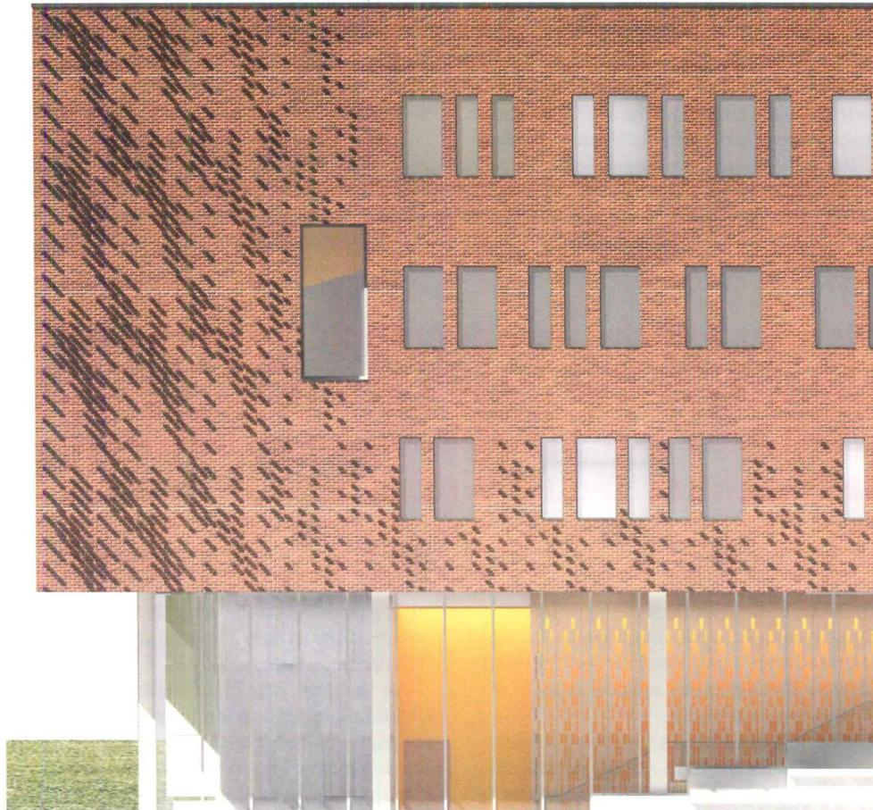
**BRICKS AND BYTES** For the facade of the Institute for Data Science at the University of Rochester (left), KVA is turning bricks perpendicular to the wall and cantilevering them at various depths (below).
