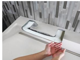
Innovative “all-in-one” handwashing fixtures include touchless functions of soap dispensing (left), water washing/rinsing (center), and hand drying (right).
