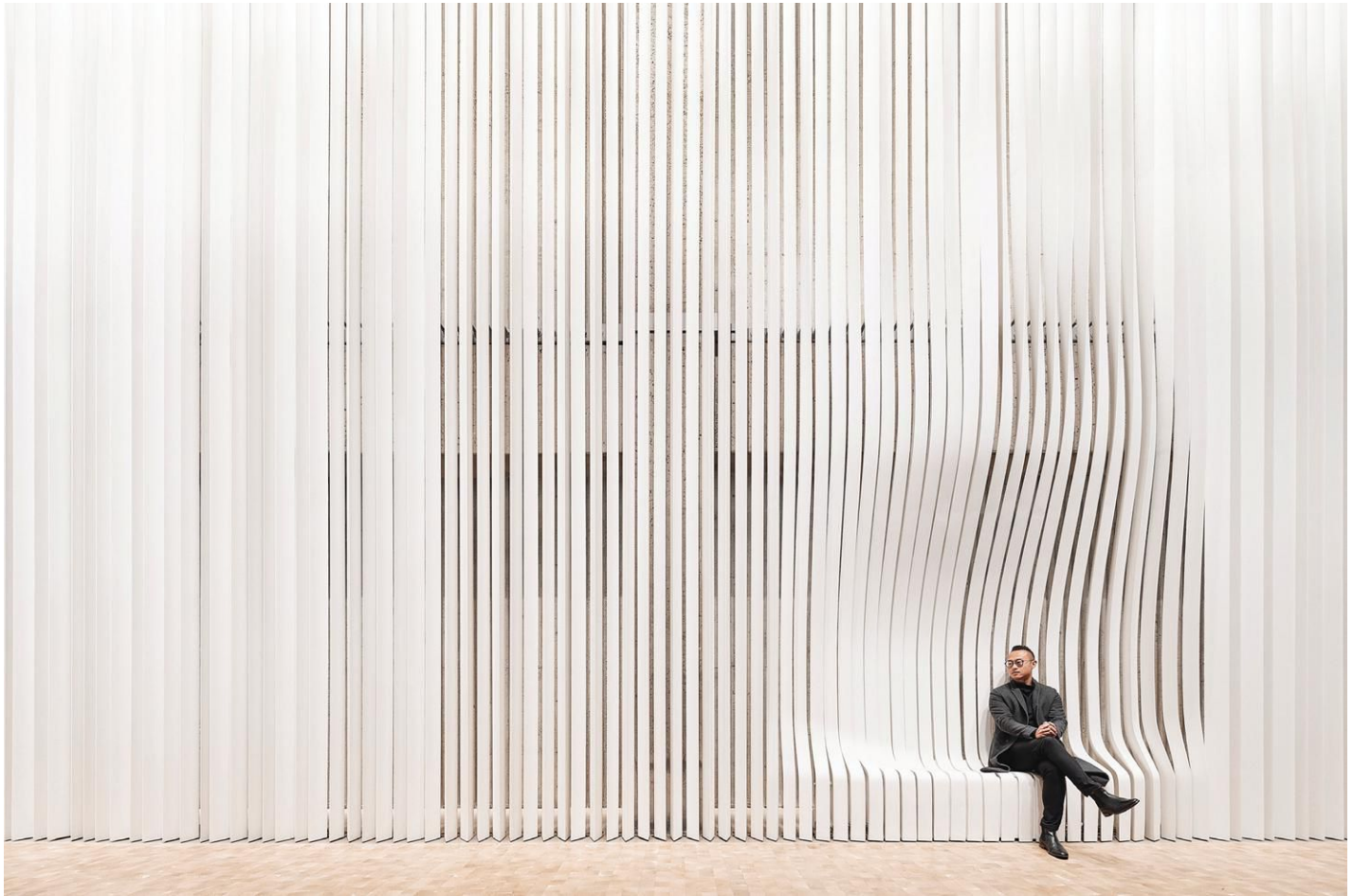
THE CURVACEOUS ribbons, triangular in plan (below, center and right) are spaced about 1 inch apart, allowing glimpses of the core and its columns and beams beyond (above). Though each of the 230 undulant elements appears unique, there are only about 20 distinct shapes (below, left).
