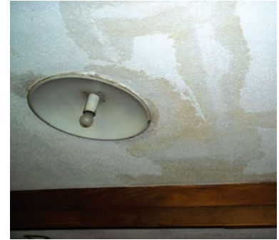
Water-damaged asbestos popcorn ceiling
