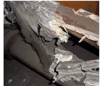
Damaged air cell insulation on pipes
