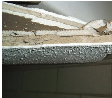
Asbestos spray ceiling on plaster
