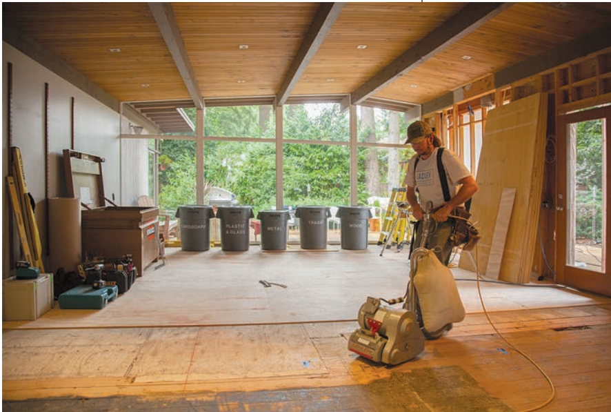
Lead carpenter Grant Kasten is sanding high spots to receive AC plywood underlayment (the 'A' side is sanded and smooth) for the terrazzo. The bag on the sander captures almost all of the dust, making a protective face mask unnecessary.
