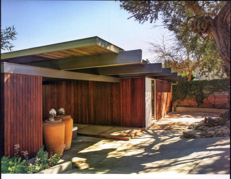
(ABOVE) THE CLASSIC POST-AND-BEAM STRUCTURE OF THE HOME HAS REDWOOD SIDING, AS IT'S THE BEST WOOD TO PROTECT AGAINST MOISTURE, ROT AND TERMITES IN THE SOUTHERN CALIFORNIA ENVIRONMENT. THE ORIGINAL TONGUE-AND-GROOVE PLYWOOD HAD TO BE REPLACED DUE TO ROT, SO RICK AND FRANCESCO TOOK ADVANTAGE OF THE UPDATE AND ADDED AN EXTRA REDWOOD PANEL WHERE THERE WAS ONCE ONLY A POST (SEEN TO THE LEFT).
