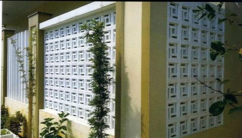
Breeze blocks can be stacked into walls that deflect rain, allow for ventilation and provide both privacy as well as outside visibility.
