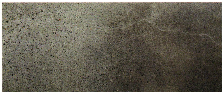
(BELOW) THE HOME'S ORIGINAL CONCRETE SLAB WAS GROUND, DIAMOND-POLISHED, STAINED AND SEALED, REVEALING BEAUTIFUL AGGREGATE COLORS AND NATURAL VARIATIONS.
