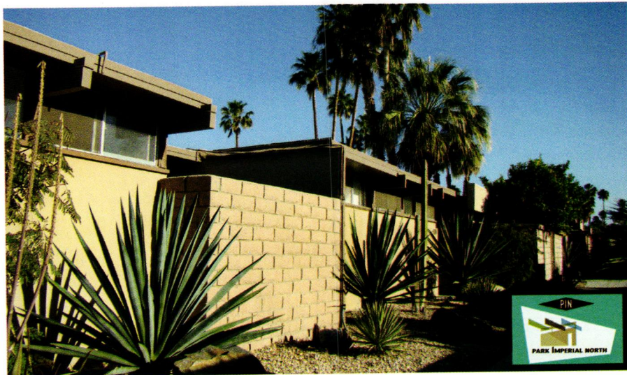
TOP: THE MOST RECENT RESTORATION PROJECT WAS THE COLORFUL ACRYLIC PANELS ON THE EAST POOL PAVILION. ABOVE: "PARK IMPERIAL NORTH IS A PERFECT EXAMPLE OF THE POST-AND-BEAM CONSTRUCTION OF MODERN LIVING, WITH ITS SIGNATURE EXTERIOR BEAMS ALLOWING A WALL OF WINDOWS ON EACH UNIT," BERGE SAYS.
