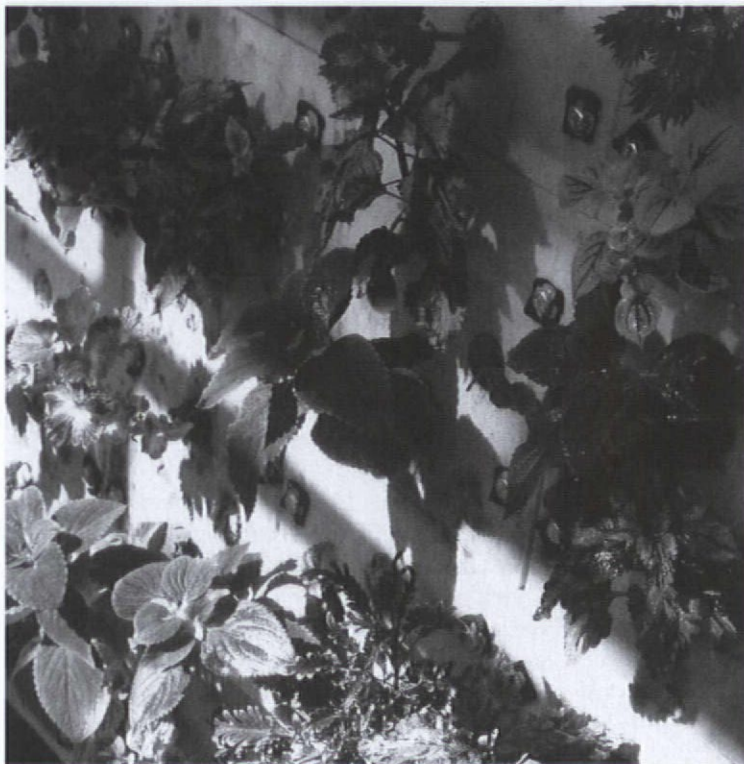
EnVitrum's structural masonry, made from 95% recycled glass, supports plant growth by enabling the movement of water through capillary action. Photo: EnVitrum
