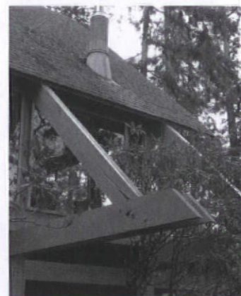
The exposed rafters and joists of the A-frame design have led to rot issues around bolted joints. Photo by Dale Kutzero
