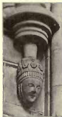
FIG. 64.—LICHFIELD CATHEDRAL. Vault-corbel in north transept.
