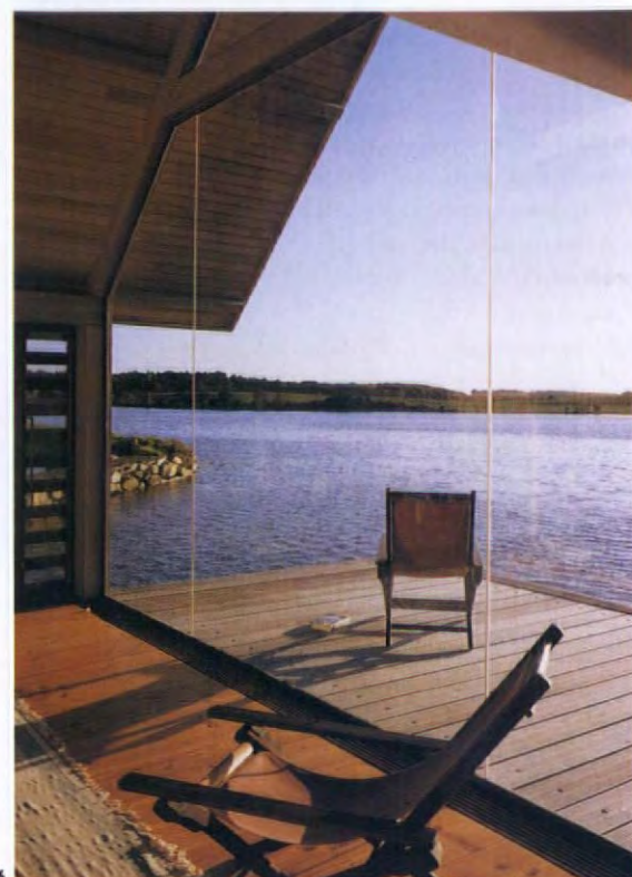
6 West wall of glass panels butt-jointed with translucent mastic.
