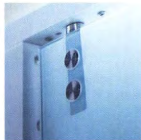
Top pivoted doors enable minimal stainless steel strips instead of large, unsightly metal patches.
