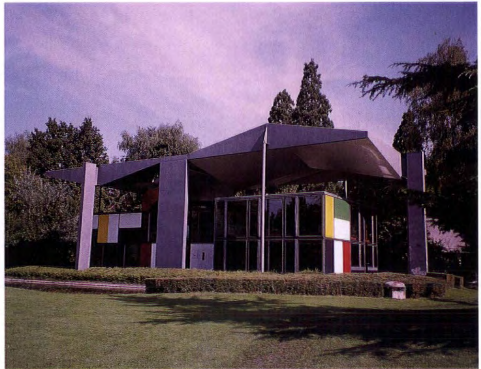
Centre Le Corbusier exhibits his sculptures and graphic works – his last and only steel-frame building.
