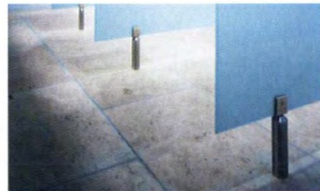
CNC turned stainless steel feet. Bolted into the floor and set out of sight 200mm. back from front of cubicle.
