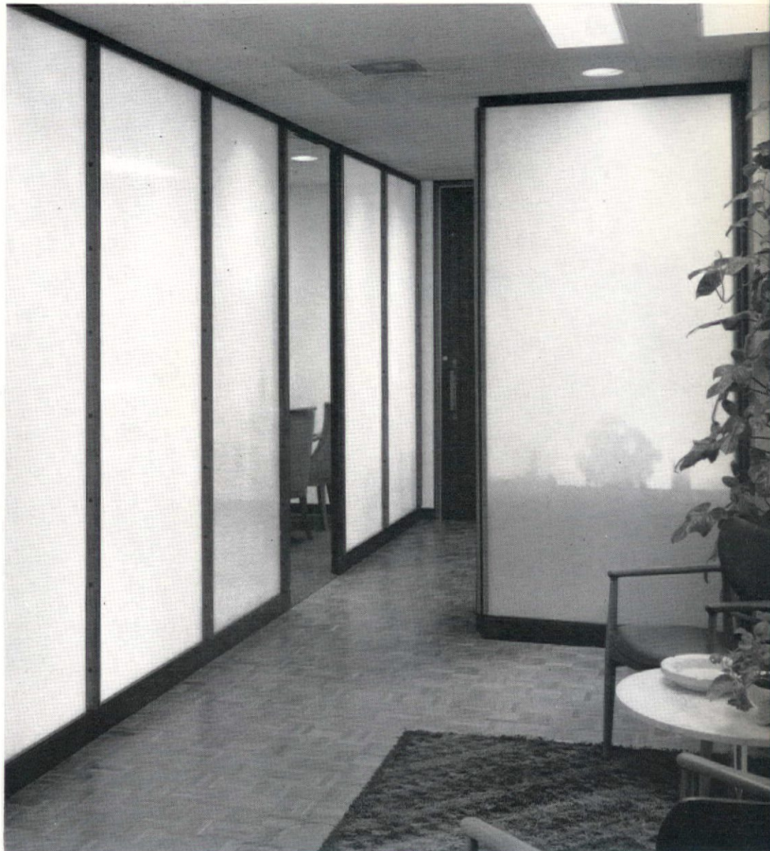
TRANSLUCENT PARTITIONS of Huewhite evenly diffuse interior illumination. Pure white of glass sets off handsome polished woods: posts are cherry with rosewood plugs, parquet floor is of cherry strips.
