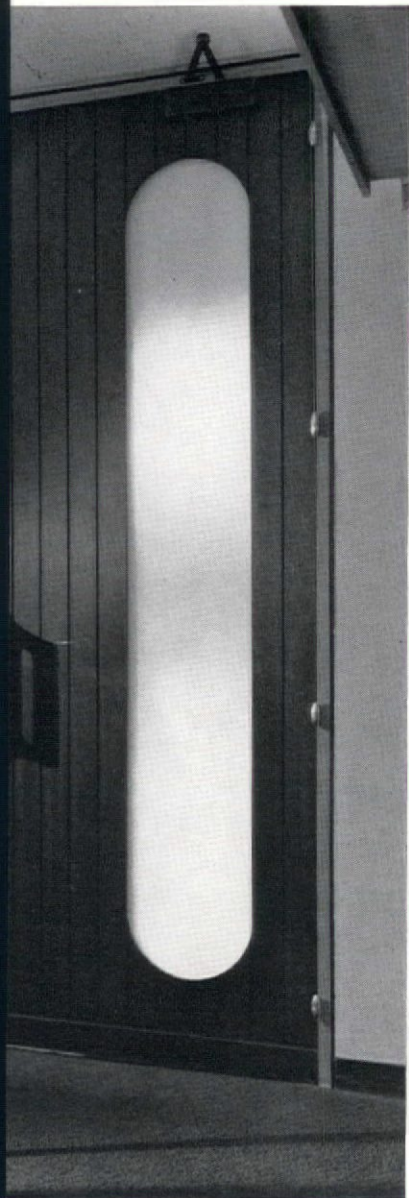
ROSEWOOD DOOR with Huewhite panel brings light from corridor into windowless board room. Glass is inserted through slot in top of door.
