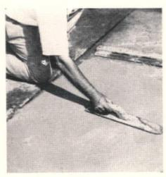
A new concrete floor resurfacer by Monroe Co. may be applied to wet or dry surfaces, indoors or out. It is self-bonding and needs no primer. The non-slip surface is trowelled directly onto deteriorated concrete at depths as thin as 1/8 in. by available maintenance personnel. Circle No. 168.
