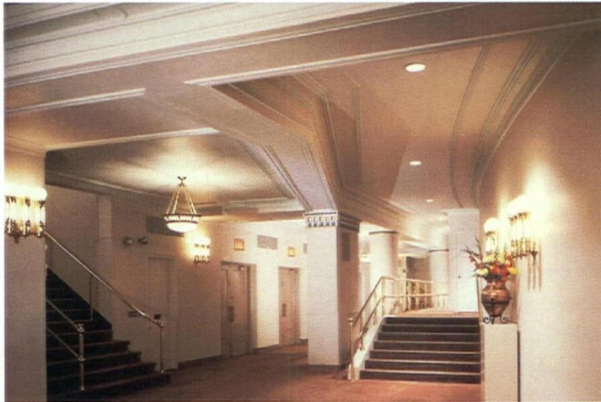
A new inner lobby (above) emerged at City Center Theater, New York, when the architects steepened the inadequate slope of the orchestra—causing it to run out of head room before reaching the rear wall and creating space for the lobby. The reconfiguration of the ceiling was accomplished through the use of both painted wood moldings and cast molding.
