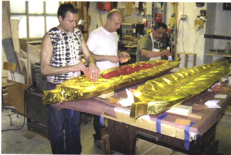
Two artisans apply gold leaf to the historic molding of the ballroom in the Prince George Hotel in New York City during a renovation by designer Jamie Drake (above left, photo courtesy of Alpha Workshops). The ceiling of the Prince George ballroom contains a painted canvas medallion (above right, photo courtesy of Benjamin Moore/ Tim Proctor Photography). Gilded carved leaves representing "totems to life" were created for Lifetime TV (below left, photo courtesy of Alpha Workshops, and below right, photo by Andy Washnik - CORPRICOM).
