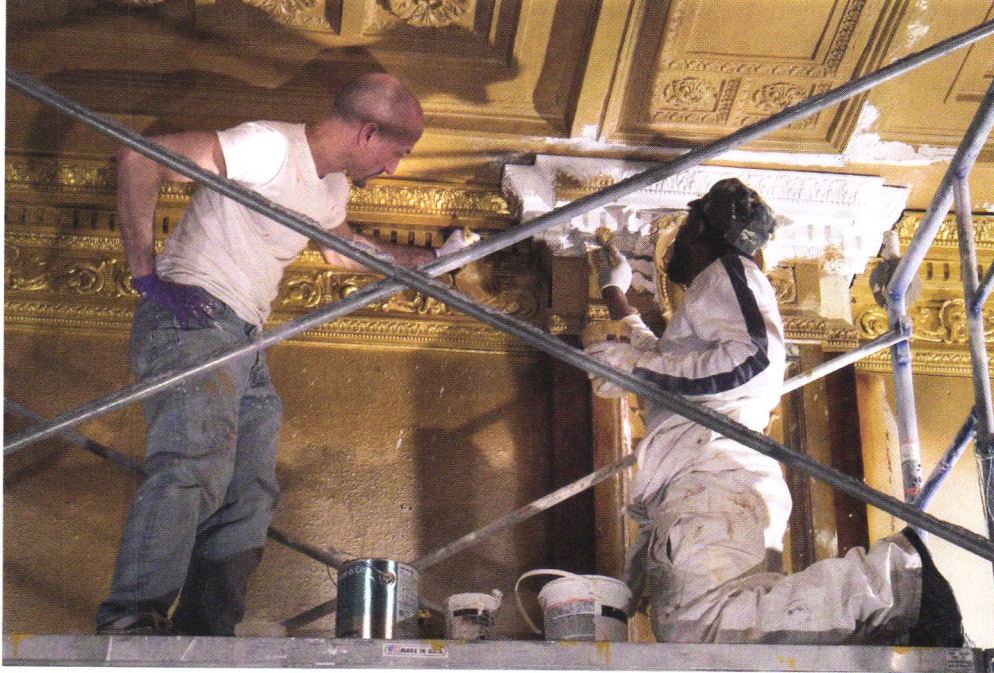
Two artisans apply gold leaf to the historic molding of the ballroom in the Prince George Hotel in New York City during a renovation by designer Jamie Drake (above left, photo courtesy of Alpha Workshops). The ceiling of the Prince George ballroom contains a painted canvas medallion (above right, photo courtesy of Benjamin Moore/ Tim Proctor Photography). Gilded carved leaves representing "totems to life" were created for Lifetime TV (below left, photo courtesy of Alpha Workshops, and below right, photo by Andy Washnik - CORPRICOM).
