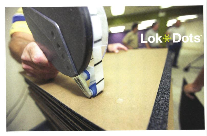
LokDots is a revolutionary adhesive for the installation of EcoWorx® backed modular carpet. LokDots is an odorless, virtually VOC-free adhesive, making it ideal for occupied space environments. LokDots also make it possible to install carpet tile in spaces with higher moisture levels on the slab compared to industry standard liquid adhesives.
