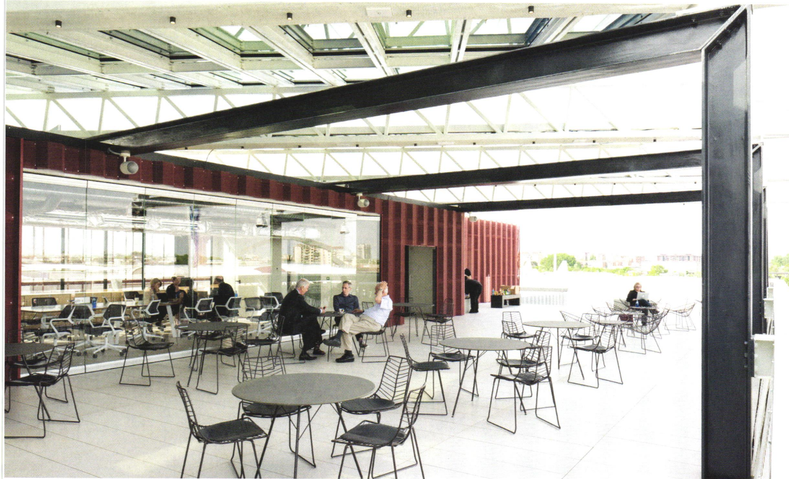
A canopy over the roof deck (above) is made with panels of Isoclima-manufactured smart glass so that the pavilion's organizers can customize the level of opacity and harvest daylight. The canopy also provides sun and rain protection for visitors.
