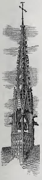
Fig. 1.--Lead-Covered Bell Turret, Minorite Church, Cologne, 14th Century. Crockets of Beaten Lead.
