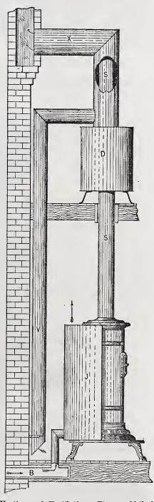
Heating and Ventilation.—Fig. 9.—Method eating and ventuation.—Fig. 9.—Method of Ventilation where Flue Opening is in Sczon- Story. B, Supply of Outside Air. V, Ventilating Pipe. S, Stove Pipe. J, Jacket to Stove. D, Drum, Located in Second Story. X, Jacket to Stove Pipe, by which the Air Withdrawn from Lower Properties Semental Hotal before Estating Room is Somewhat Heated before Entering Chimney Flue.
