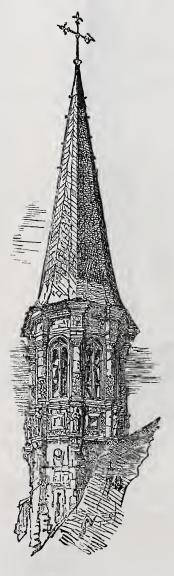
Fig. 3.-Bell Turret of Stone, with Pinnacle of Wood Covered with Slate, 16th Century.
