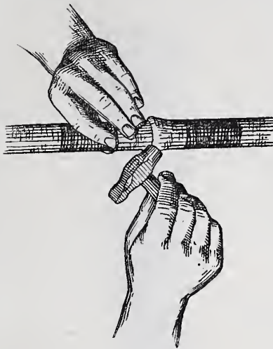
Plumbers' Joints.—Fig. 6.—Uniting the Ends of Lead Pipe Preparatory to Making a Wiped Joint.
