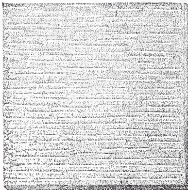
Fig. 4.—Pane Ax Granite Work.
