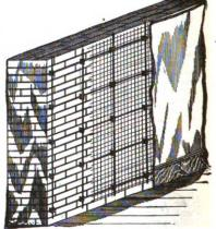
Fig. 3.-Lathing as Applied to Brick Walls.
