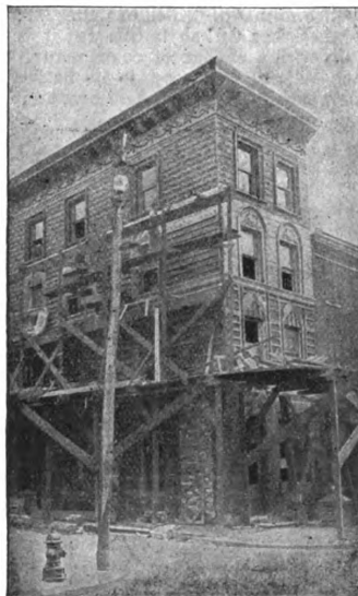
Fig. 4.—Putting on the Metal Plates.
