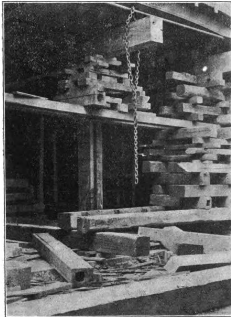
Fig. 2.—View Showing Timbering and Temporary Blocking.
