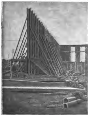
Fig. 4.—Bracing Used in Constructing West Wall of Round House.
