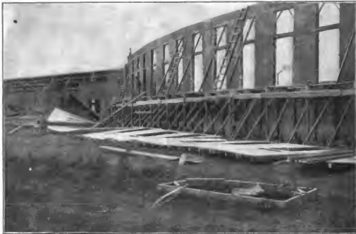
Fig. 3.—Exterior of Round House Walls, Showing Wooden Frames Used in Construction.
