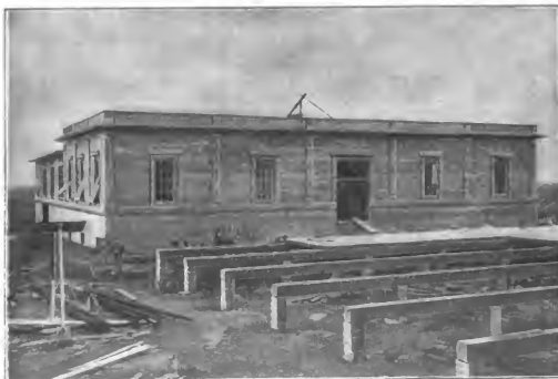
Fig. 5.—The Power House, Built Entirely of Concrete.
