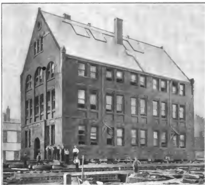
Fig. 1—General View of the Building as it Appeared During the Operation of Moving.
