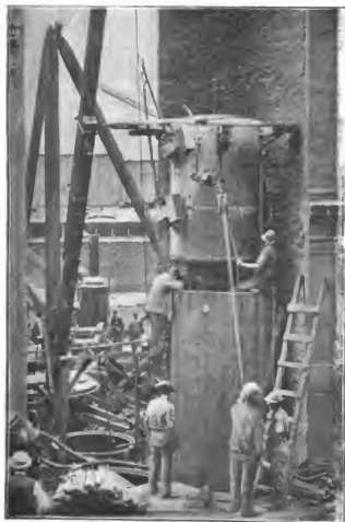
Fig. 5.—Circular Caisson with its Air Lock.
