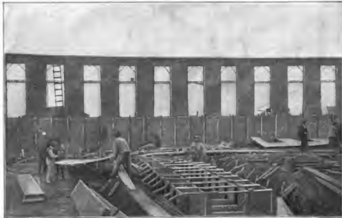
Fig. 2.—Interior of Round House. Wooden Boxes in Foreground are Molds for Concrete Track Beds.
