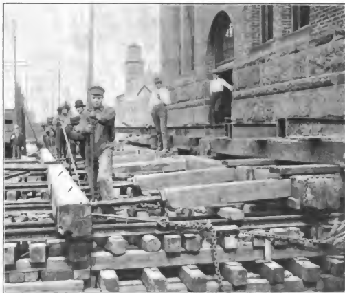
Fig. 2—View Showing the "Shoving Screws" and the Patent Hook for Taking Up Slack in the Chains.
