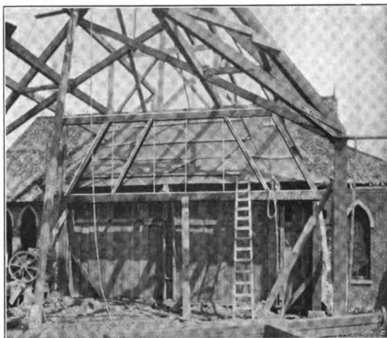
Fig. 2.—Showing Truss Supporting Old Roof of Lecture Room.
