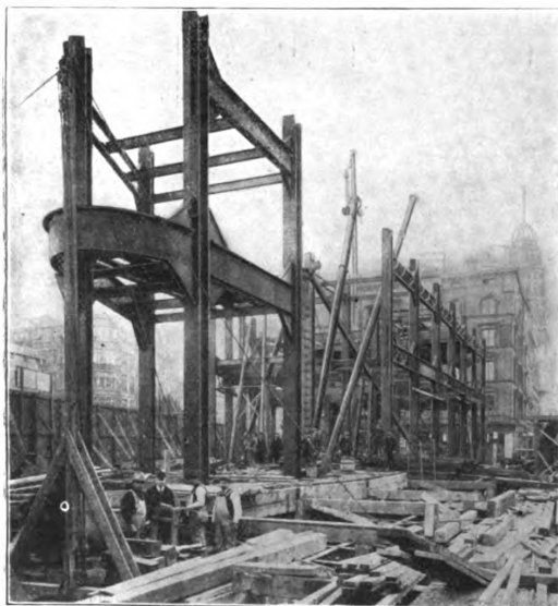
Fig. 1.—View of the Framing of the Rounded Apex of the Triangle as it Appeared March 10.
