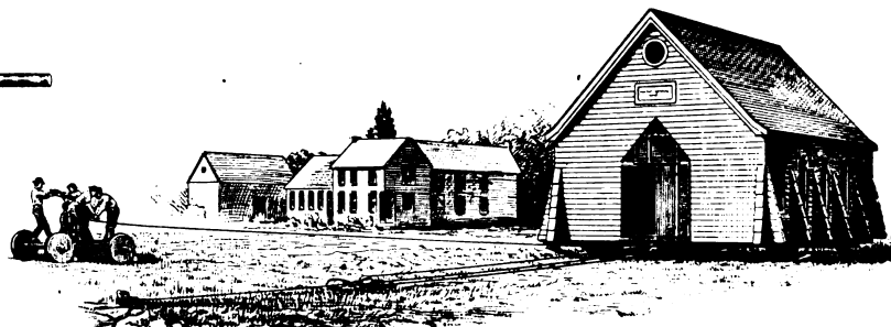
Fig. 5.—Method of Moving Light Frame Buildings.
