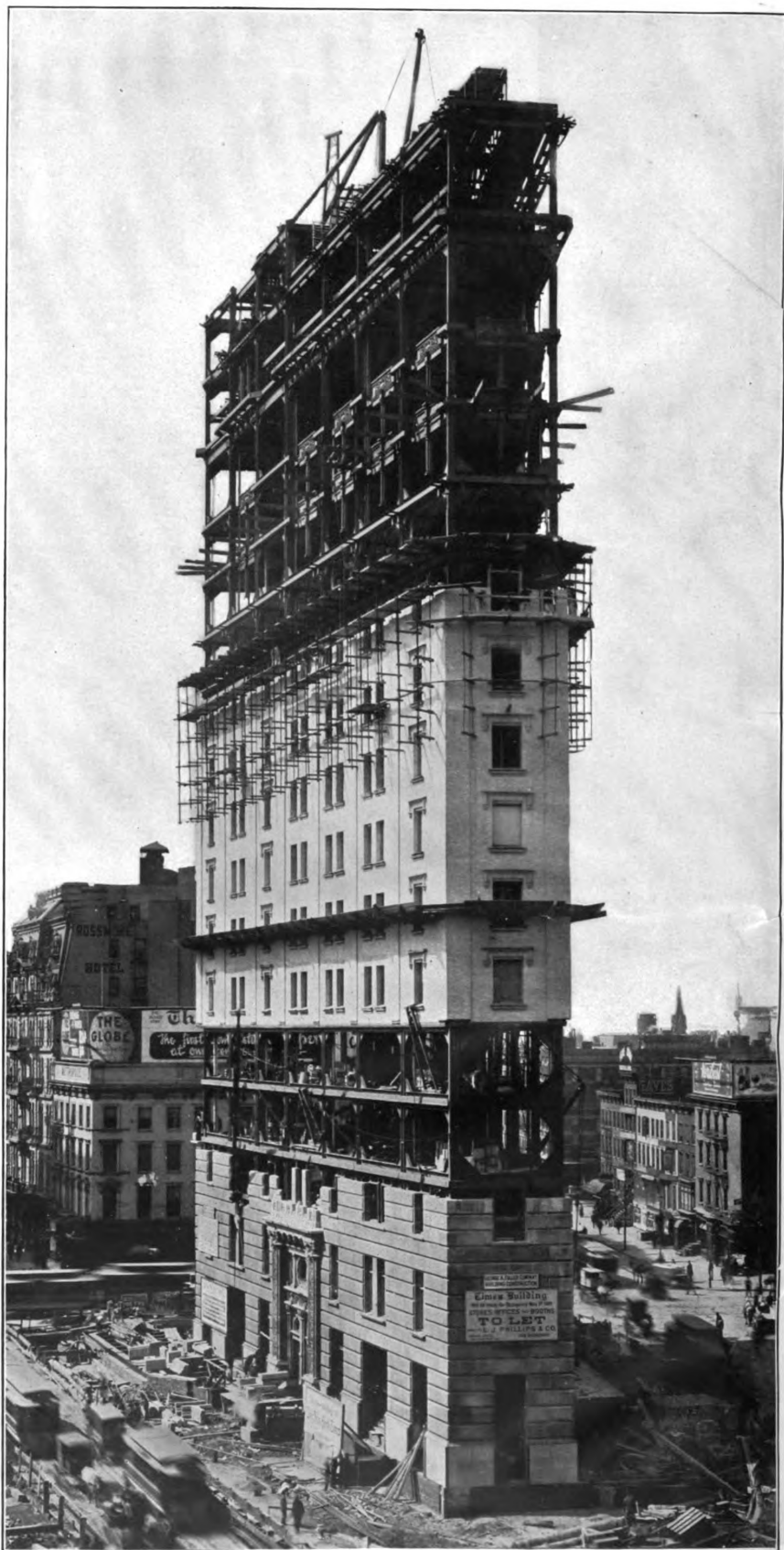
THE "NEW YORK TIMES" BUILDING AS IT APPEARS IN PROCESS OF ERECTION.
