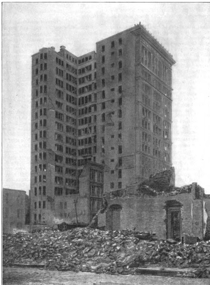
View of Rear of Continental Trust Company's Building, showing the brick wall which was so seriously damaged that it will have to be taken down. The cause of the injury was the method of construction; metal ties being used for bonding the bricks.
