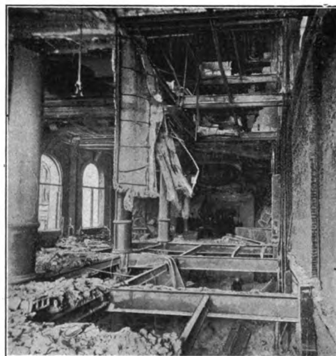
Fig. 4.—Interior View of the Equitable Building, Showing Where Floor Arches Have Fallen.
