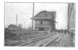
Fig. 1.-Building Ready to Be Loaded on Cars.
