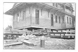
Fig. 2.-View of Corner of Building After Being Loaded on Cars.
