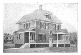
8 ft. 4 in. and the cellar 7 ft. Across the front and part way on one side is a piazza, the lattice work underneath being hung on hinges in order to facilitate putting the coal in the cellar. The porch columns are of the Tuscan order.
