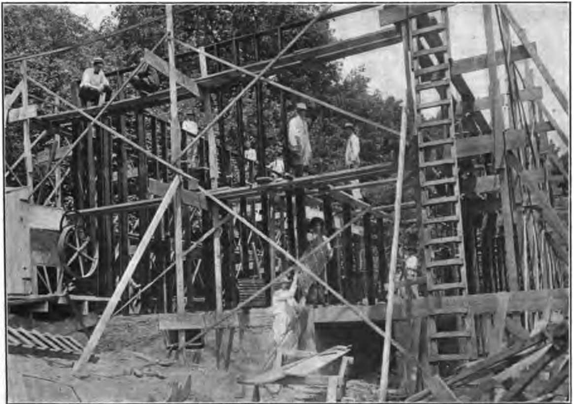
View Showing Method of Erecting the Studding of the Building by Means of a Scaffold Extending Around the Exterior of the Structure.
