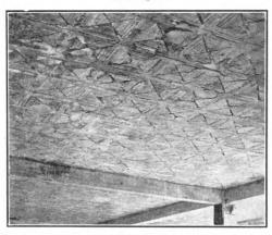
Fig. 4.—Appearance of Ceiling After Floor Is Laid and "Centering" Removed.
