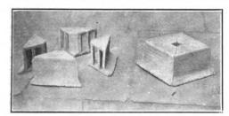
Fig. 1.-View of a Block or Tile and Its Component Parts.
