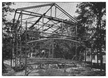
Fig. 1.-View of Skeleton Frame Made of Steel Tubing.
