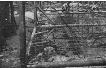
Fig. 2.—Showing the Horizontal Truss System,
