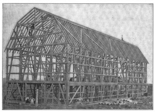
Perspective of Plank Framing Ready for the Outside Board Covering.
