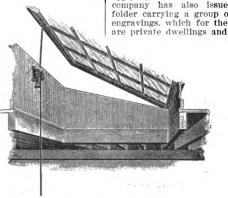
Fig. 9 .- The Payson Skylight Operator in Use.
