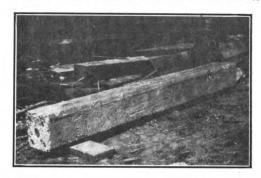
Fig. 5 .- Concrete Pile with Ends Cut Off Square Ready for Test.
