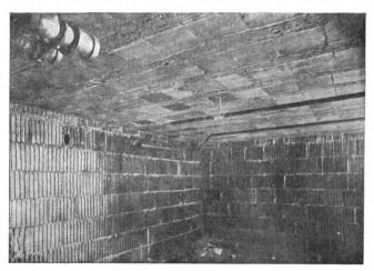
Fireproof Houses.—Fig. 1.—Interior of a House in Newark, N. J., Showing a Tile Bearing Wall with a Typical Floor Resting on It.
