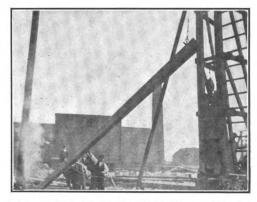
Fig. 2.—Pile Being Pulled Into Place, the Hammer Being Down to Steady Machine.
