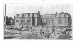
Fig. 3.—Side View of Building While Being Moved Toward the Left.—A Portion of the Old Cellar Is Seen in the Foreground.
