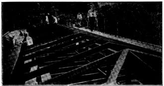
A Metal Lumber Dwelling in process of construction. Metal Rafters and Sheathing being put in place
