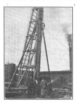
Fig. 3.—The Pile in Position and the Machine Ready to Begin Driving.
