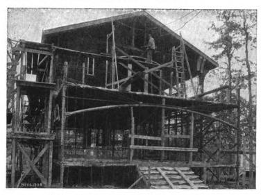
Fig. 4.—Applying the Cement Plaster on the Outside Walls.
