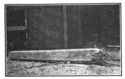
Fig. 4.—Pile with Head Smashed, Exposing Reinforcement.
