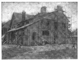
Fig. 5.—House Showing Exterior Stucco Work in Process.
