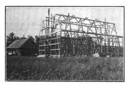
First Plank Frame Barn in Arcadia, Mich.—Fig. 1.—Side View of Frame Before Rafters Were in Place.—Cabin of Pioneer Built in 1868 Shown at the Left.
