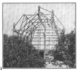
Fig. 2.—End View of Frame Showing Concrete Basement
