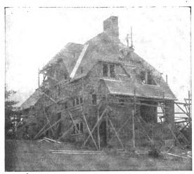
Fireproof Houses.—Fig. 3.—House in Course of Construction, Showing Concrete Foundations and Method of Setting the Tile.
