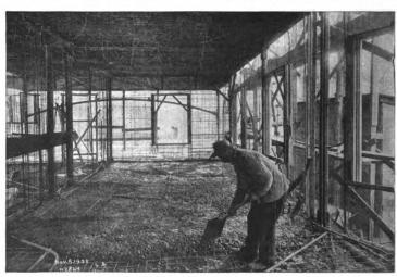
Fig. 3.- Placing the Concrete on the Floor.
