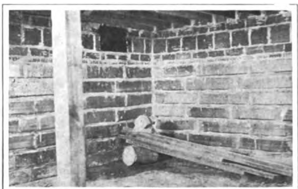
CORNER OF THE BASEMENT SHOWING CONDUITS AND THE HOLLOW WALLS LAID UPON THEM
