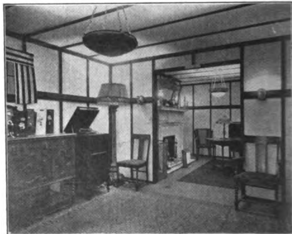
Fig. 6—Showing Use of Neponset Wall Board in Connection with Exhibition Booth Construction
