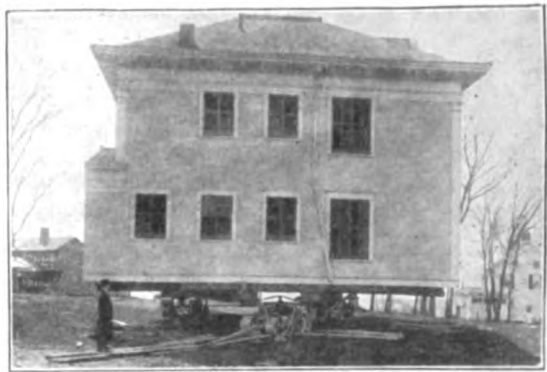
Fig. 2—A 12-Room House Loaded on the 3-Point Method
