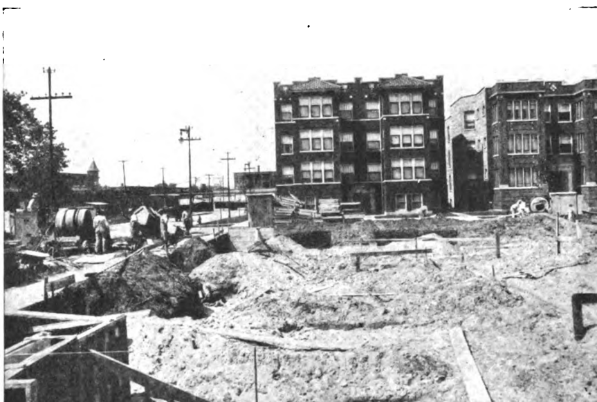
Economy Methods in Concrete Foundation Work—Fig. 3—View of "Standard" Low Charging Mixers on the Job
