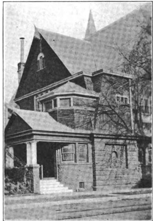
Fig. 26—Rear View of Fig. 25, Showing Shingled Cornice
