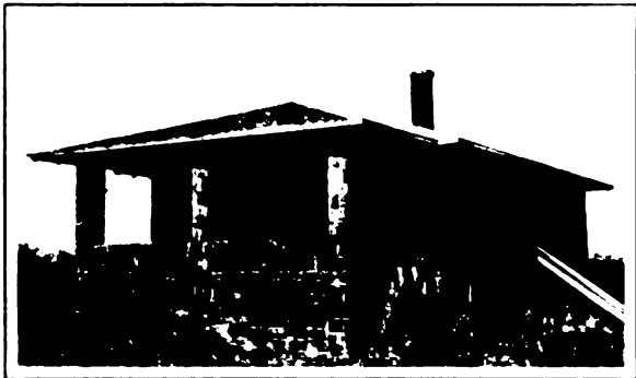
Building a Modern Low Cost Bungalow of Hollow Tile Construction—Porch View Before Stucco Was Applied
