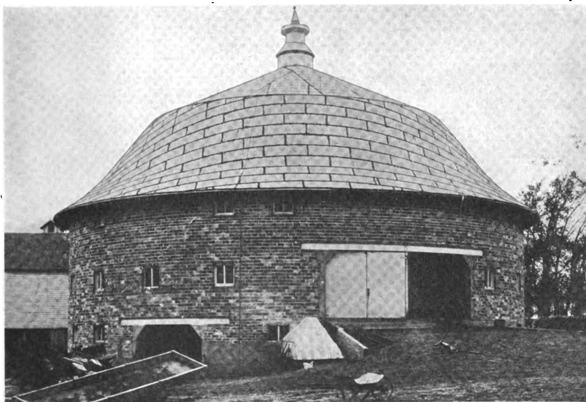
Fig. 1—A Good Example of Round Barn Roofed with "Transite" Asbestos Shingles
