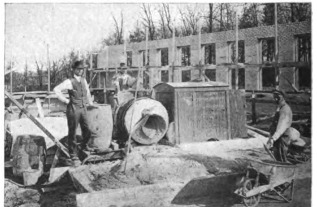
Fig. 9—Another View of the Building Operation Showing the Mixer
