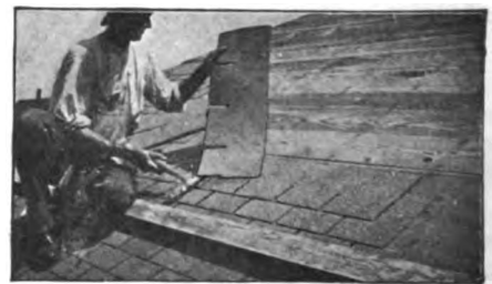
Fig. 13—Another View of the Laying of Rex Strip Shingles
