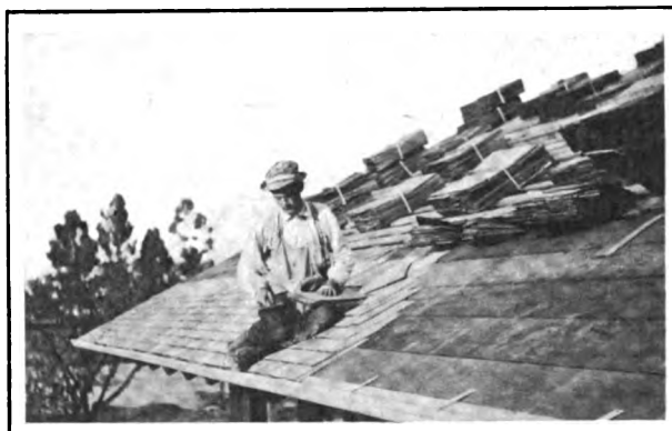
Fig. 16—Method of Holding the Shingles by the Workman
