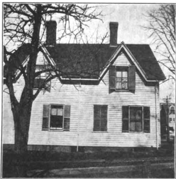
Fig. 3—House Showing Tops Tipped Away from Each Other
