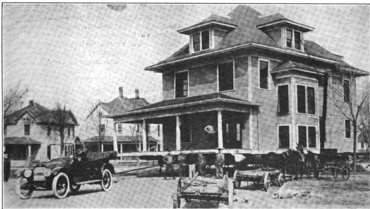
Moving a Two-Story and a Half Frame House by Means of an Automobile
