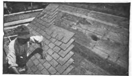
Rex Roofings and Shingles—Fig. 12—Laying Rex Strip Shingles
