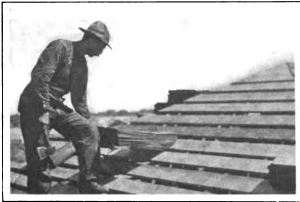
SOME ASPECTS OF MODERN SHINGLING. FIG. 4—PUSHING THE LOWER ROWS OF THE BUNDLE IN BETWEEN ROOF BOARDS
