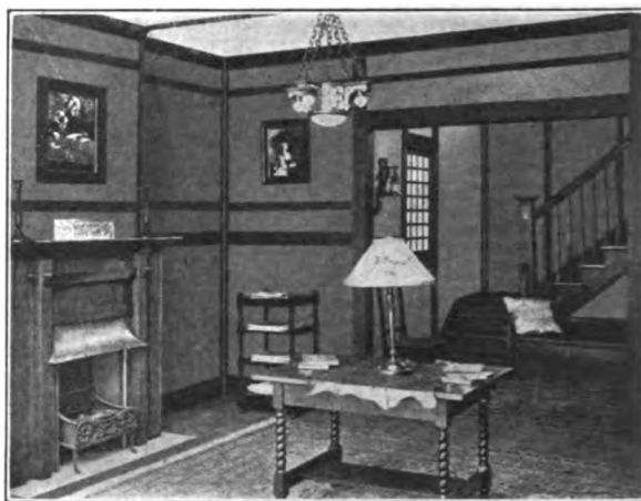
Fig. 8—Showing Application of Black Rock Wallboard as an Interior Finish
