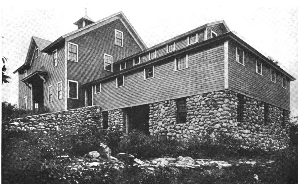
VIEW OF COMBINATION BARN, SHOWING THE FIELD STONE FOUNDATION AND THE RETAINING WALLS
