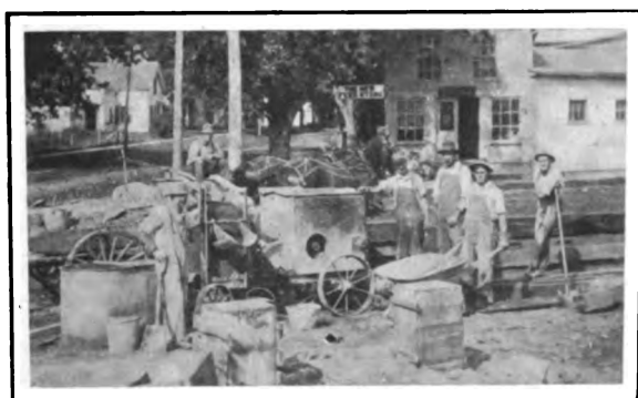
A Small Portable Concrete Mixer in Use in Connection with a Suburban Job
