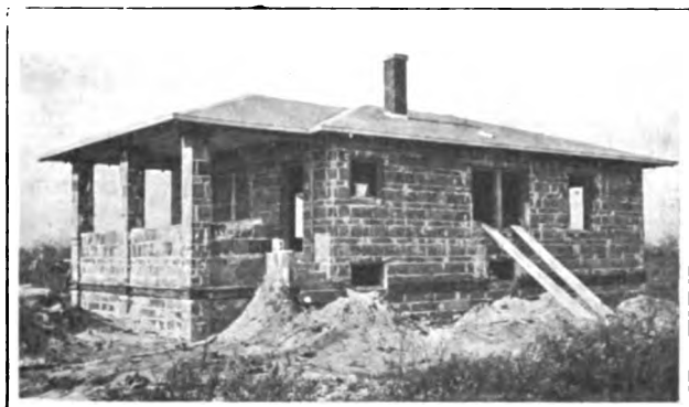
THE SOUTH SIDE OF THE HOUSE BEFORE THE EXTERIOR COATING OF STUCCO HAD BEEN APPLIED
