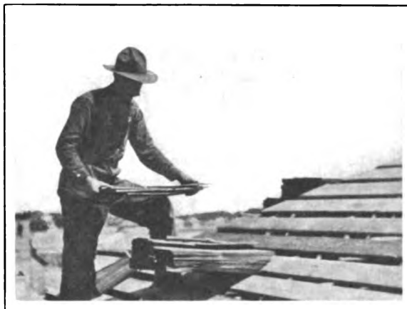
FIG. 5—THE NEXT STEP IN DISTRIBUTING THE SHINGLES
