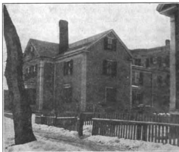
Fig. 4—Chimney Showing Bend Over the Narrow Side
