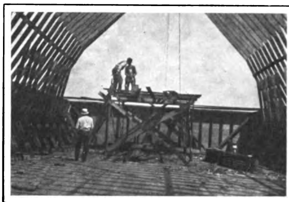
Inside View of the Framework Showing the Temporary Working Platform
