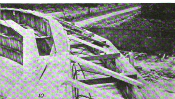
"PROGRESS" PICTURES SHOWING DIFFERENT STAGES OF THE CONSTRUCTION WORK ON THE ROUND REINFORCED CONCRETE BARN
