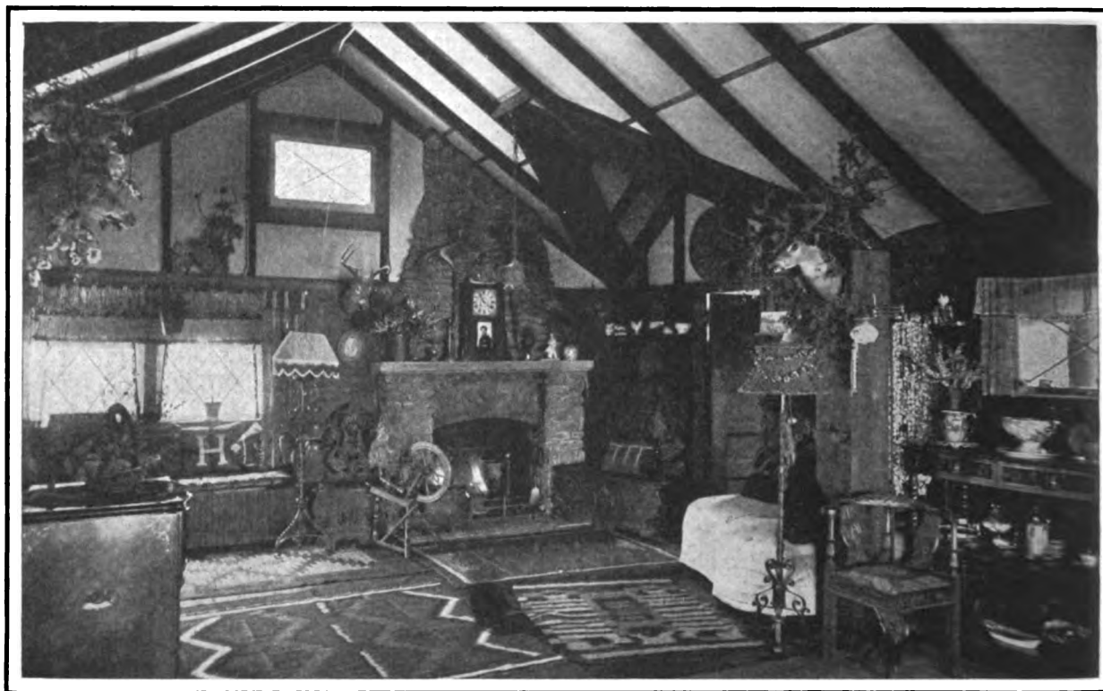
Fig. 4—Living Room of a Cottage at Atlantic Highlands. Showing Ceiling and Side Walls Covered with Wall Board
