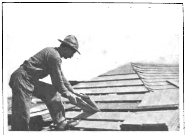
FIG. 6—PUSHING THE TOPS BETWEEN THE ROOF BOARDS
