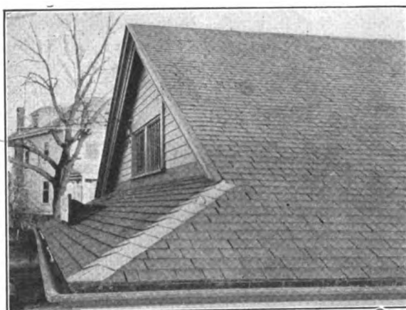
Fig. 36—Appearance of the "Boston Hip" on a Roof
