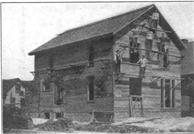
"Trouble Saver" Building Brackets in use
