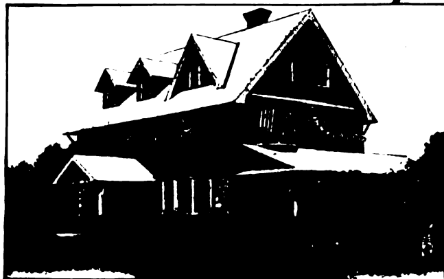
Residence of D. T. Dickson, Wayne, Pa. Covered with J-M Transite Asbestos Shingles Francis T. Gugert, Architect, Wayne, Pa.
