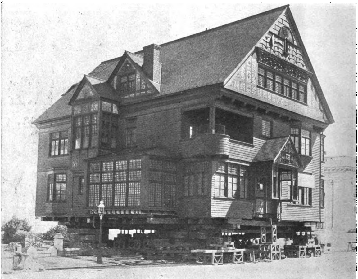
A VIEW OF THE BUILDING AFTER IT HAD BEEN RAISED FROM ITS FOUNDATIONS
