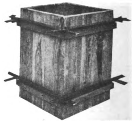
Fig. 10—The Mims Clamp for Concrete Forms
