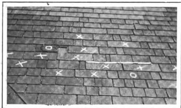
Some Aspects of Modern Shingling—Fig. 17—Showing That Wide Shingles Do Not Always Split After Laying
