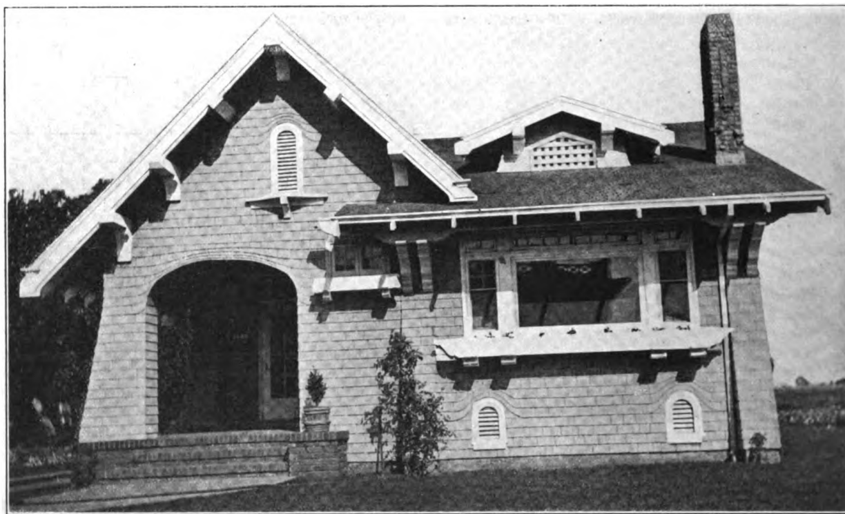
Fig. 51—A Good Example, Showing Appearance of Shingling Around Curved Openings
