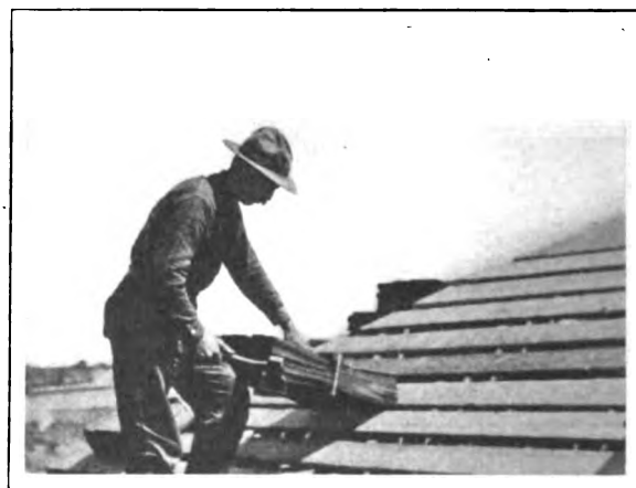
Fig. 3—Opening a Bundle of Shingles Preparatory to Beginning Work
