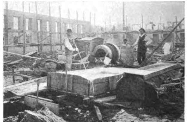
Concrete Mixers for Mortars and Plasters—Fig. 8—The Machine in Use
