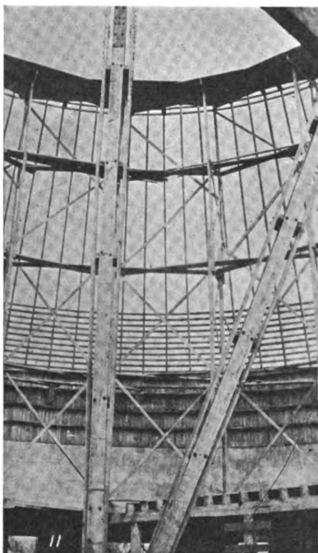
"PROGRESS" PICTURES OF THE FIRST ROUND REINFORCED CONCRETE BARN ERECTED IN THIS COUNTRY
