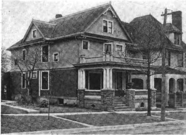
A STUCCO COAT FOR THE SECOND STORY
