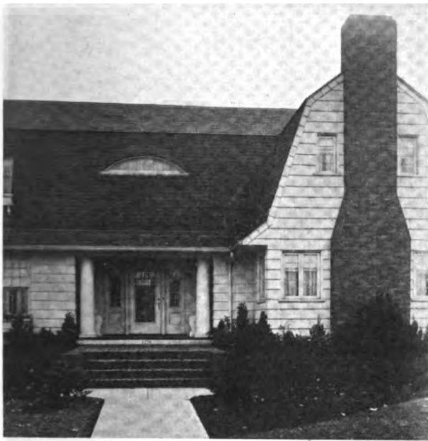
DETAIL OF FRONT ENTRANCE AND SHOWING THE OUTSIDE CHIMNEY
