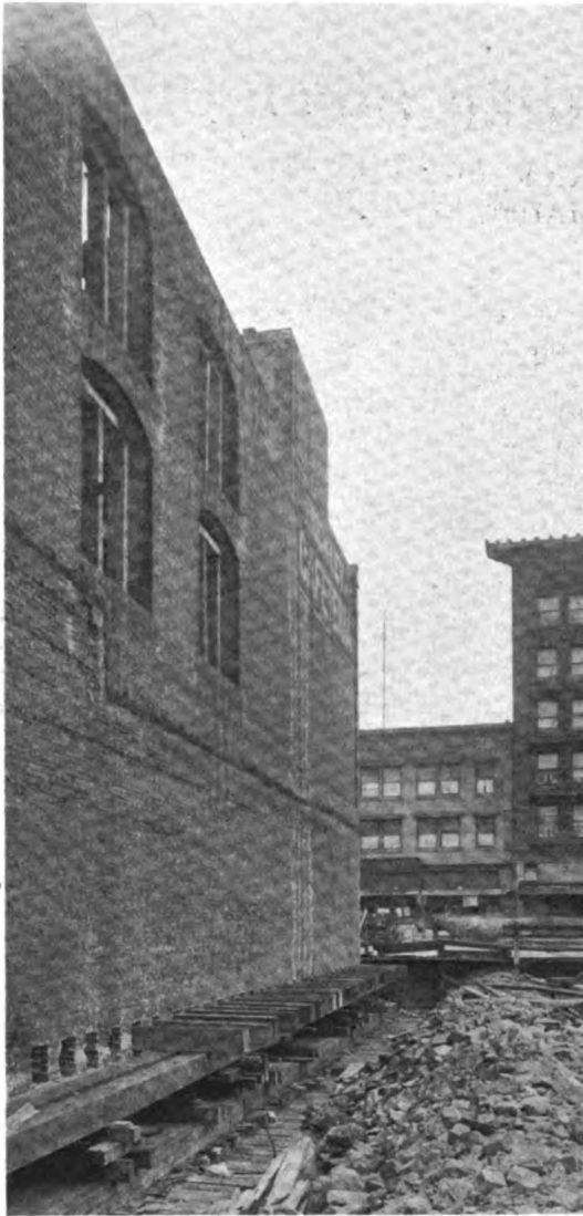
FIG. 2—SIDE VIEW SHOWING HEIGHT OF THE BUILDING TO BE MOVED
