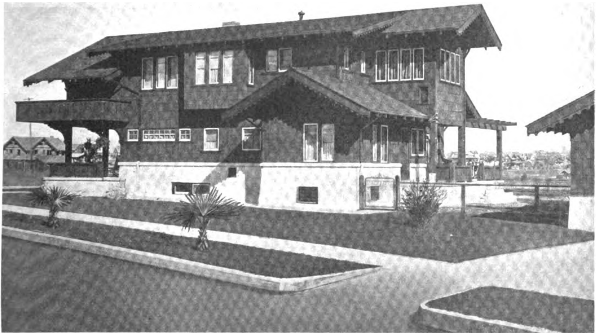
SIDE AND REAR VIEWS OF CHALET BUILT BY A. S. BARNES AT LOS ANGELES, CAL.— PORTION OF THE GARAGE IS SEEN AT THE EXTREME RIGHT
