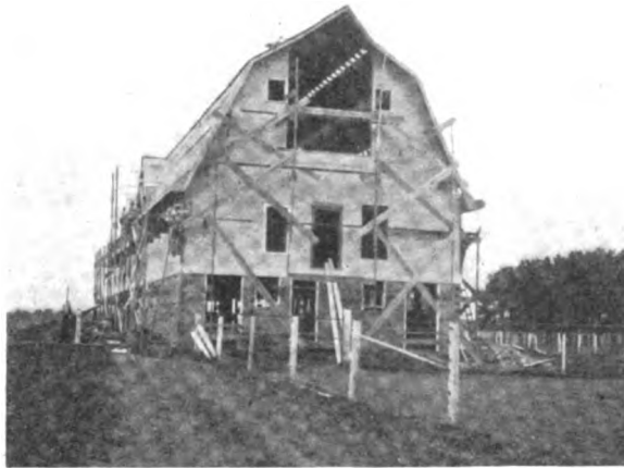
Northeast View Showing Barn During Progress of Construction
