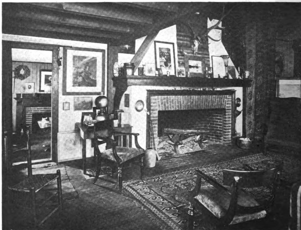
View in the Studio-Living Room of the Home of Mr. Bicknell, at Winchester, Mass.—the Open Fireplace for Burning Wood a Feature
