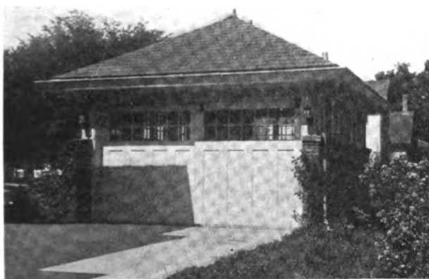
Fig. 23—Garage with Parallel Doors Closed
