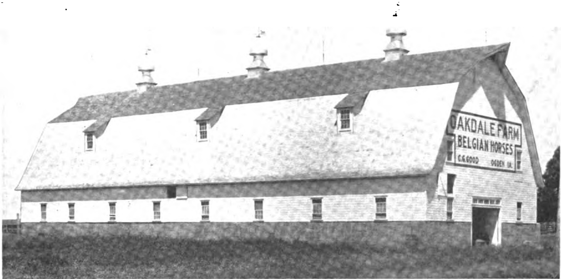
Appearance of the Finished Horse Barn on the Oakdale Farm at Ogden, Iowa
