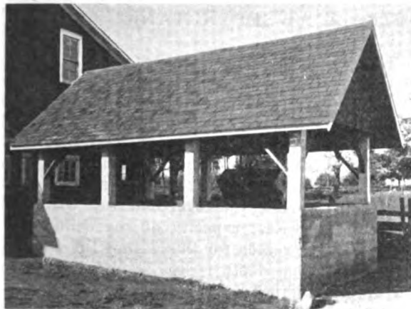
A CONCRETE MANURE PIT
