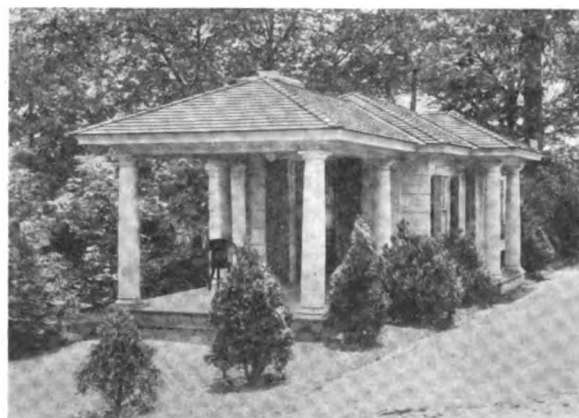
Fig. 3—View from the Left Side
