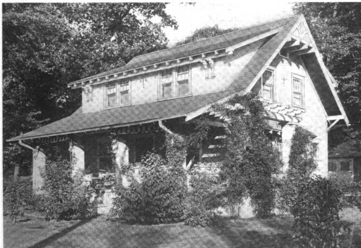
THE HOME OF M. LAWRENCE AT PELHAMWOOD, N. Y.—ARCHITECT, W. S. MOORE, NEW YORK CITY
