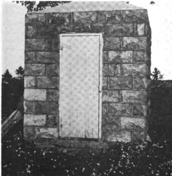
Fig. 7—A Concrete Block Smoke House with Flat Roof
