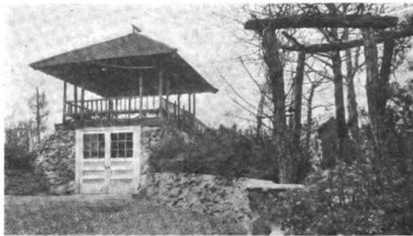
Fig. 1—Showing the Front of the Garage with Summer House on Top
