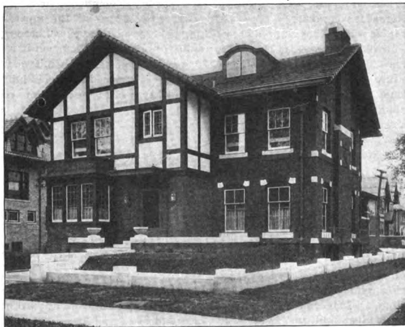
COMBINATION OF BRICK AND HALF TIMBER EFFECTS
