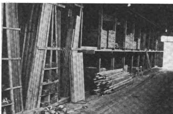
Another View of the Interior of the Shed
