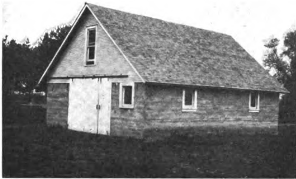
Fig. 4—Concrete Machine Shed
