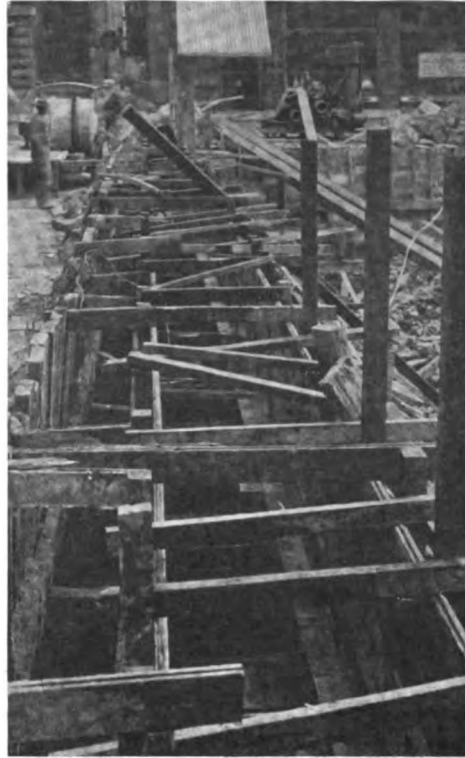
VIEW LOOKING ALONG THE LINE OF THE "FORM" FOR THE WALL
