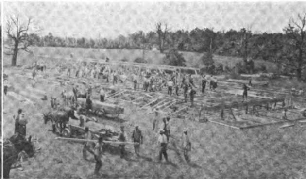
No. 4—Setting the First Floor Posts and Second Floor Girders
