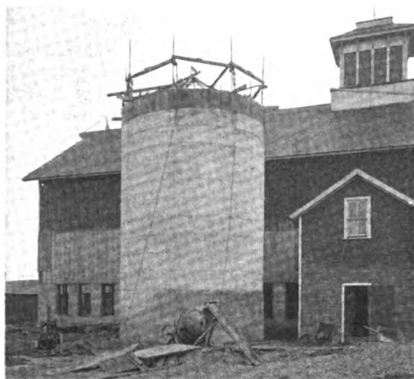
BUILDING A CONCRETE SILO
