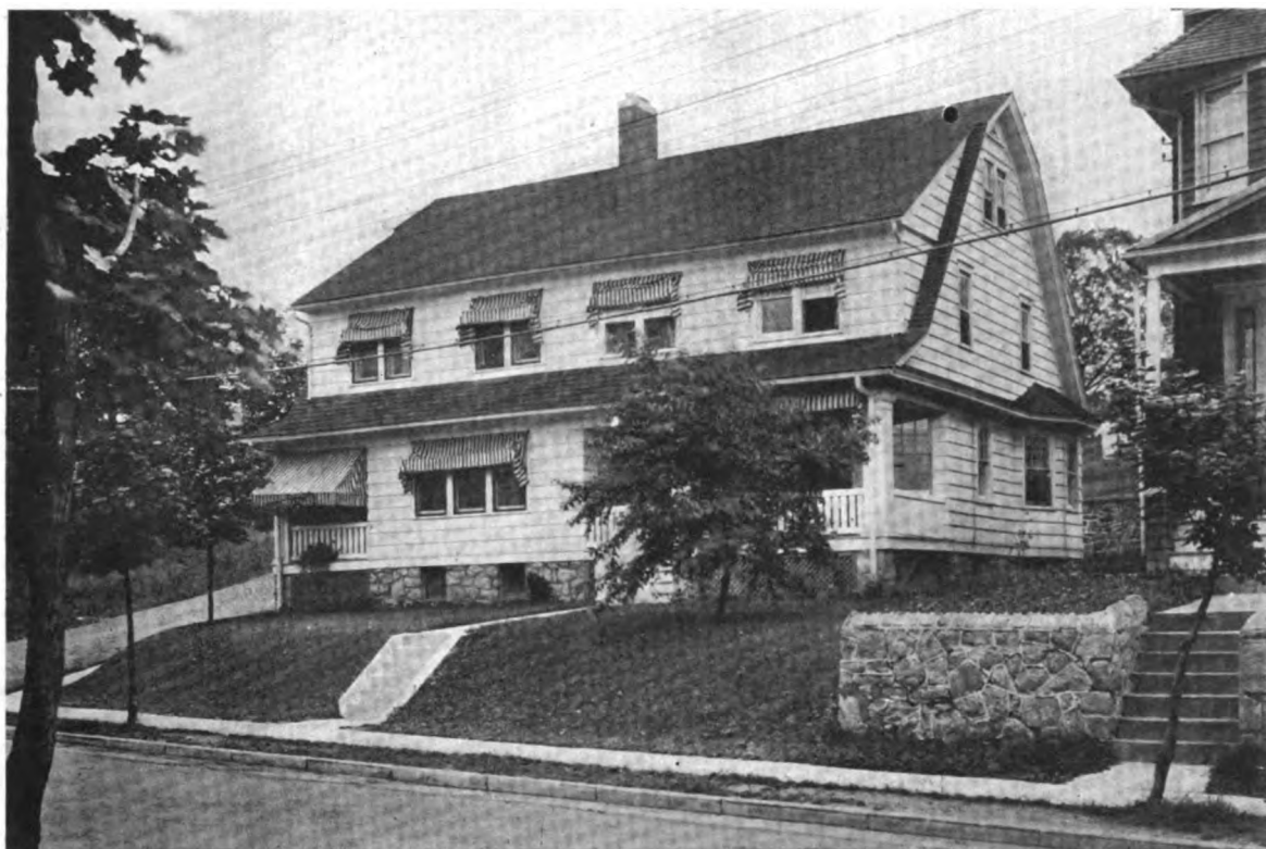
Photographic View Showing the Street Approach From One of the Main Entrances
