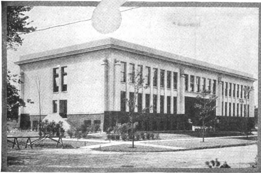
District School No. 75, Evanston, Ill. Raeder & Wood, Chicago, Ill., Architects
