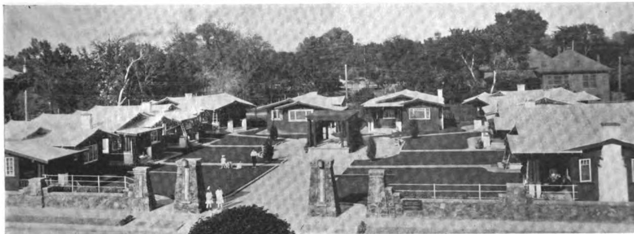
THE HINCHCLIFFE BUNGALOW COURT AS VIEWED FROM THE MAIN ENTRANCE AND SHOWING THE DISPOSITION OF THE TEN BUILDINGS OF WHICH THE COURT CONSISTS
