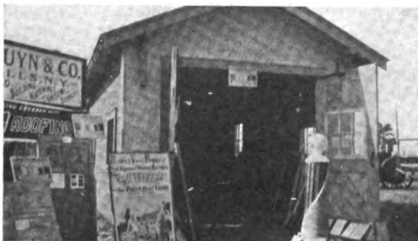
View of the Garage with the Doors Open
