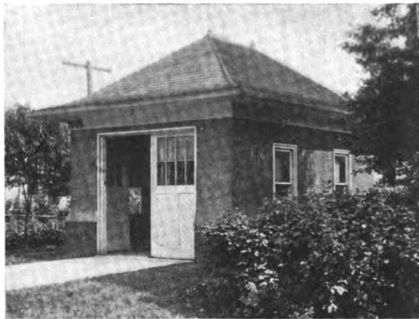
Fig. 9—The Same Garage With One of the Doors Entirely Open
