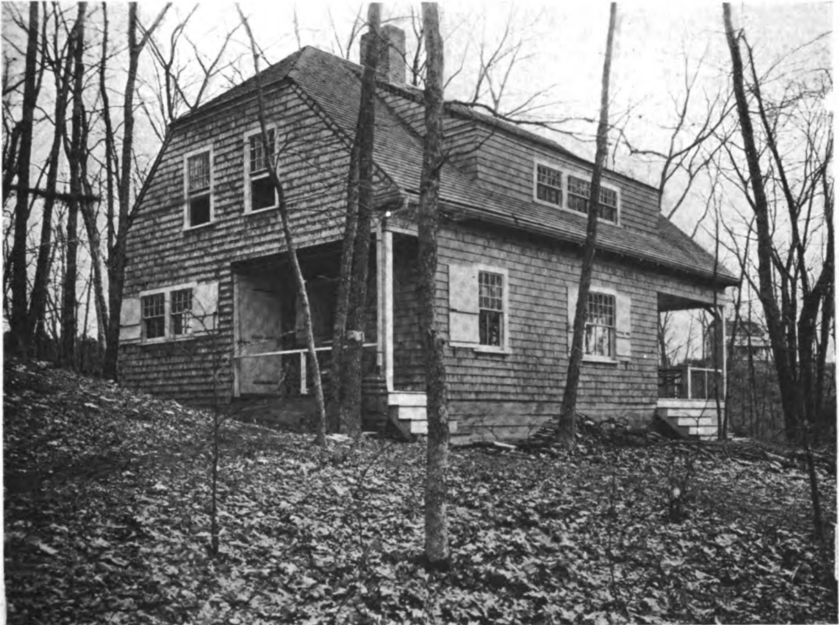
ANOTHER COTTAGE PICTURESQUELY PLACED—THE SUMMER HOME OF W. P. HUBON, LOCATED AT DANVERS, MASS.
