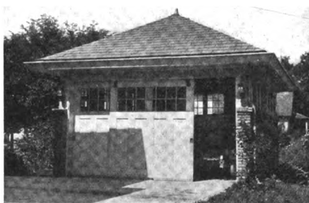
Fig. 24—Parallel Doors Partially Opened
