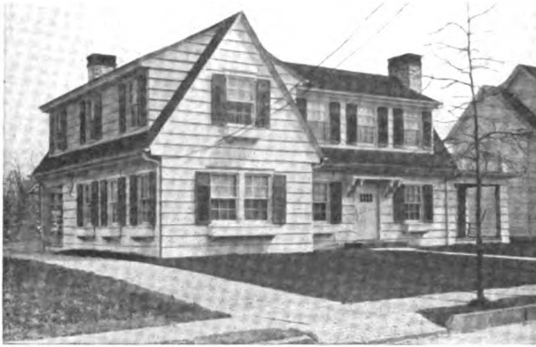
The Street Approach to the House and Showing the Left Side Elevation
