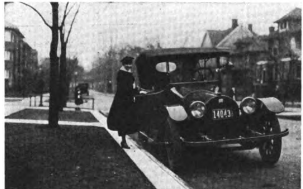
Fig. 3—Narrow Concrete Walks Along the Street Curb
