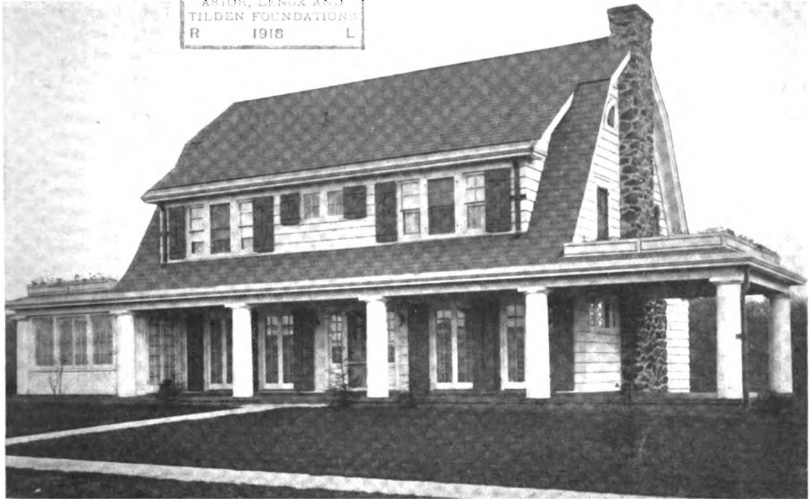
RESIDENCE OF MR. W. C. REED AT HARMON, N. Y.—ARCHITECT HENRI VALLET
