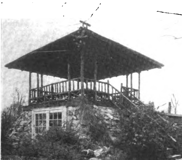
Fig. 2—Showing the Steps Leading to the Summer House
