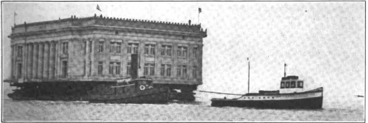
THE OHIO STATE BUILDING RESTING ON BARGES AND BEING TOWED DOWN SAN FRANCISCO BAY
