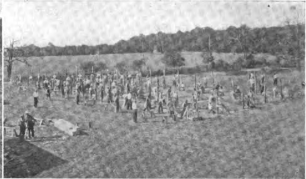
No. 2—Cutting Off the Foundation Posts
