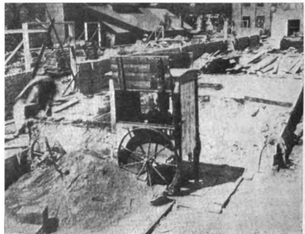
Fig. 5—Outfit for Preparing Mortar
