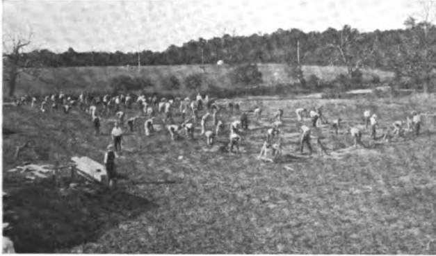
No. 1—Digging the Holes for the Foundation Posts
