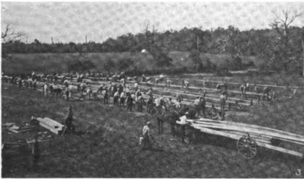
No. 3—Setting the Sills and Girders
