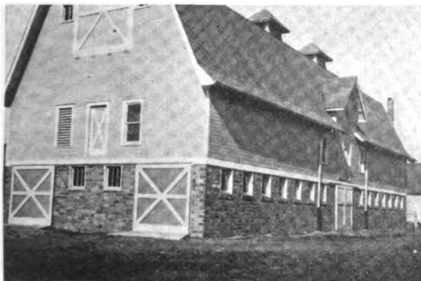
Southeast View Showing End Gable and One Side Elevation
