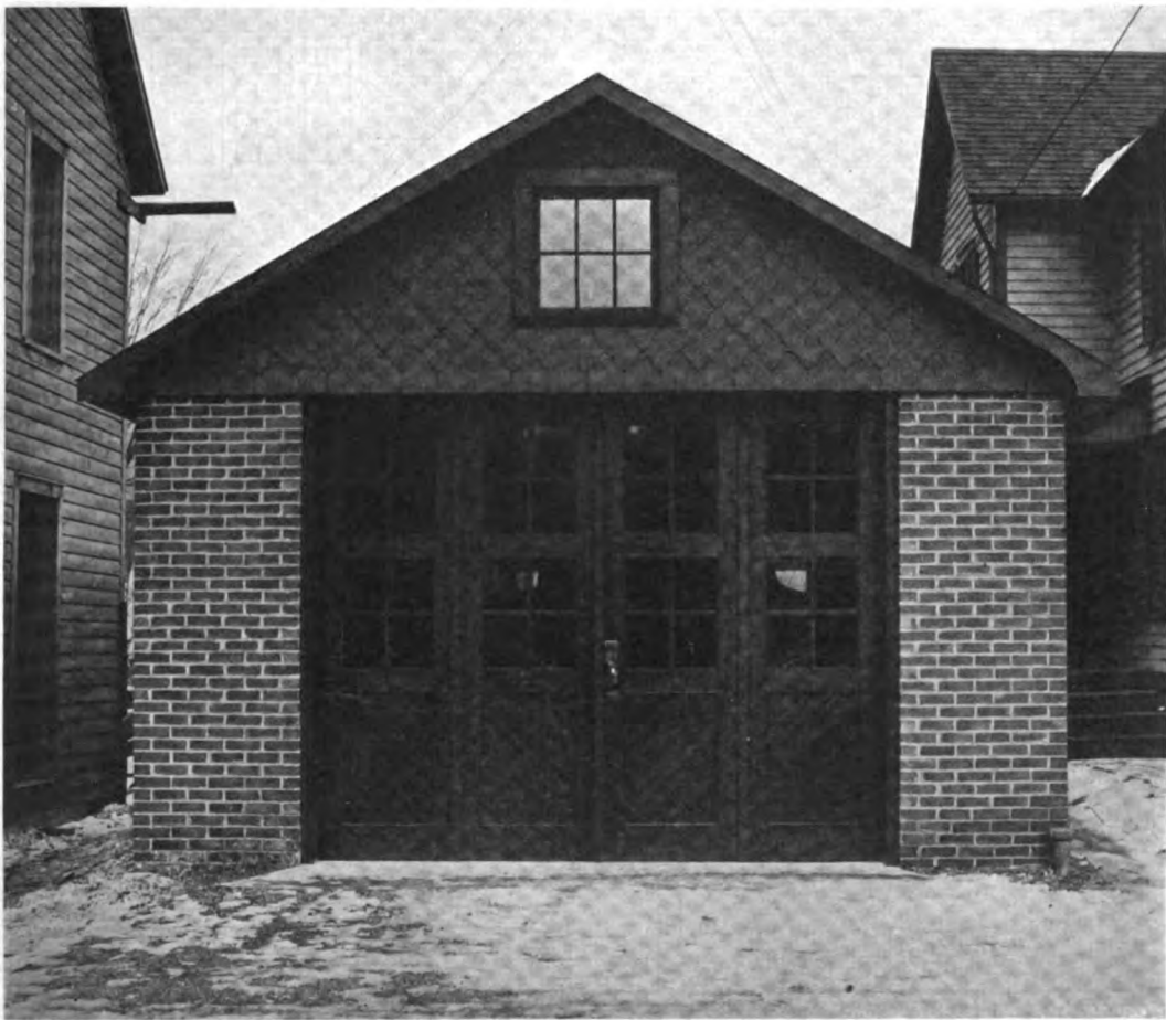
BRICK GARAGE DESIGNED AND BUILT BY WILLIAM H. WELSH, CORNING, N. Y.
