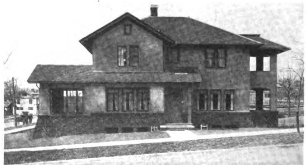
A MORE COMPLETE COAT OF STUCCO
