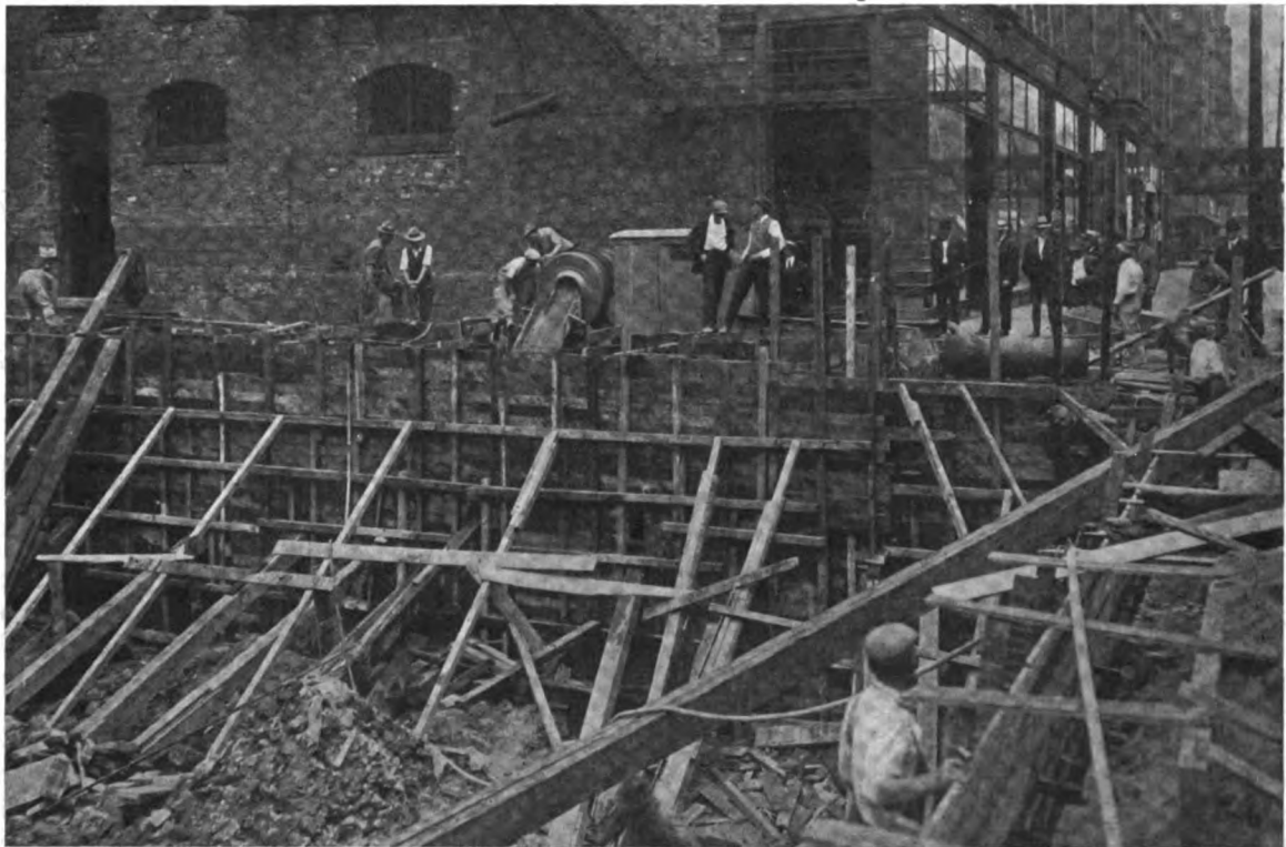
Looking Toward the Alley Where the "Forms" for the Wall Are in Place and the Concrete Is Being "Poured" Directly from the Mixer
