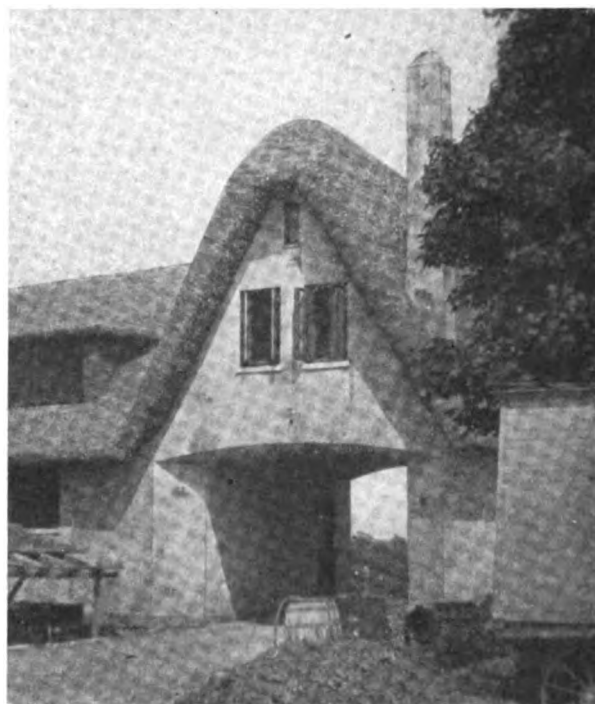
Fig. 2—Gate Lodge of S. F. Pryor Roofed with Hudson Shingles So Laid As to Give the Thatched Effect
