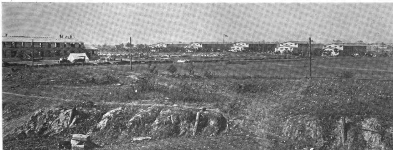
View of Section No. 1 Showing Administration Building Used During the Work of Construction as Headquarters for the Contractors and Army Officers Engaged in Building the Cantonment at Louisville
