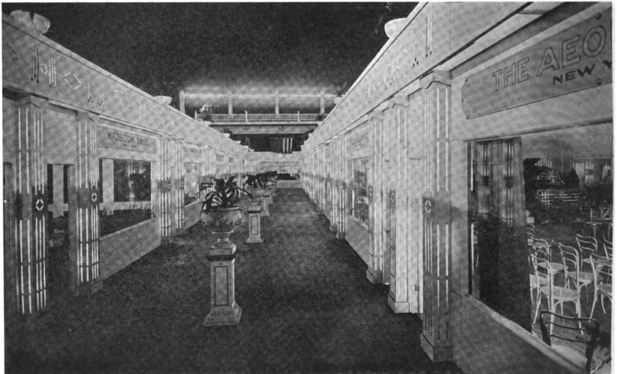
Fig. 4—View Down Aisle Toward End of Coliseum at National Music Show with Booths Constructed of Cornell Wall Board
