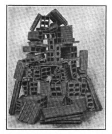
Fig. 71—Types of hollow-tile blocks made specially for fireproofing.
