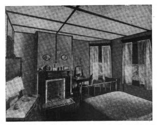
Wallboard used with battens covering wall and ceiling joints
