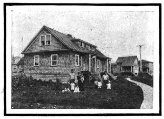
Workmen's Houses of the Standard Refractories Co., Kestler, Pa. Preventing the spread of fire is one of the biggest problems of community housing. Here it was solved by wide spacing and the use of metal roofing.
