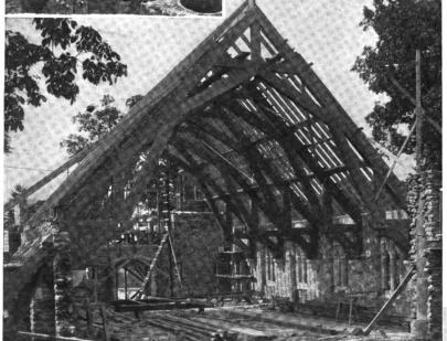
Truss of 41 ft. span for main part of church
