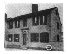
The sill here is exposed to rain, and will gradually rot
