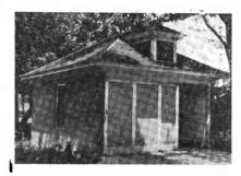
Figs. 1 and 2—A serviceable garage of hollow tile
