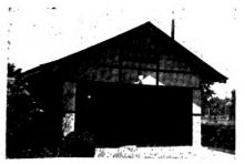
Fig. 18—An attractive frame and stucco garage, with folding doors.
