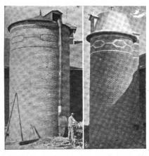
A brick silo being filled. The feed door is continuous, being made air tight by metal strips
