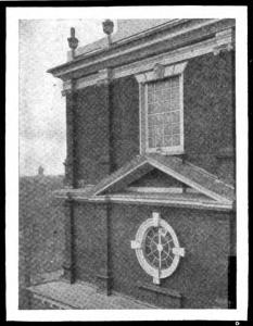
Wood Pediments and Cornices on the Tower of Independence Hall protected by Roofing Tin.
