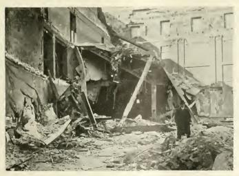
Another View of the Remaining Portion of the Balcony, Showing the Construction, the Cantilever Extended Out to the Next Twin Pilasters.
