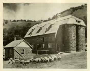
THERE are many advantages in having a barn built of other material than wood. A hollow tile barn such as we illustrate here is much warmer than a frame structure, which we too often find with wide cracks in the sheathing, affording but little real protection from the outside cold.
