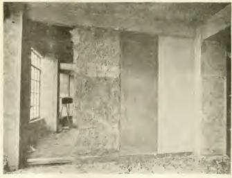
Four Different Stages in the Construction of the Plaster Partition on Jute Net Support
