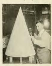
Fig. 6-Elevation of Conic Roof, Showing Method of Sheathing
