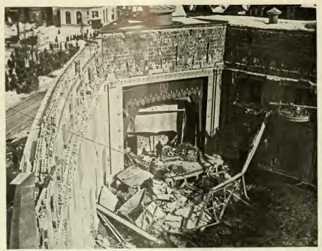
View Looking Towards Stage, Showing Wreckage of Roof and One of the Collapsed Trusses. The Hollow Tile Walls Held Up,
