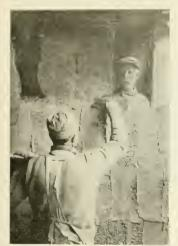
Plasterers Working Together Against Each Other on Both Sides of Jute Net Support for Plaster Partition
