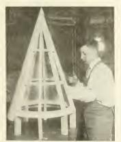
Fig. 5-Elevation of Covic Roof, Showing Method of Framing
