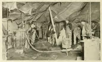
Hand mixing outfit within canvas enclosure using live steam for heating the water. A salamander heats the enclosure
