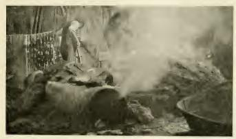
Sections of a discarded smoke stack in use on the Chicago Union Station job for heating aggregates
