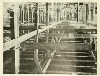
The Supporting Timbers for the Channels and Pans Note the Clamps That Hold the Removable, Upright Supports
