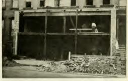
Fig. 1—The Proper Shoring and Needling Needed in Converting Two Five-story Tenements Into Stores. Observe How the Steel Breastrunner Girder is Placed to Carry the Four Upper Stories
