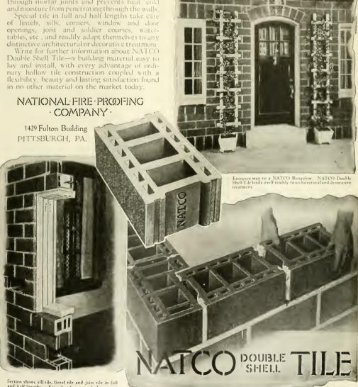
Section shows sill tile, lintel tile and joist tile in full and half lengths. Ennugh other special shapes are furnished to take care of ordinary residence details.
