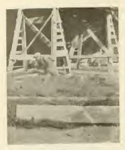
Walks and floors and other low work are Irequently protected by covering with heavy paper covered with straw, Heavy planks are used to weight the covering
