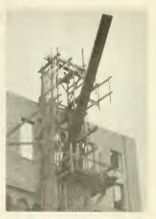
How the Steel Beam Was Successfully Raised to Top of Shalt Ready to Be Lowered Through Window
