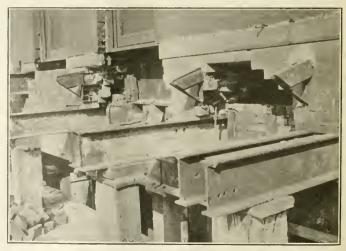
Fig. 11—The use of old steef I-beams is recommended for needles. This photo shows their use in remodelling a store front. The new steef girders are already in place and the new supporting brick work is ready to be built upon the new girder.
