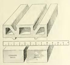
"Fisklock" is as easily handled as a common brick. It is light, and has the 4-inch hand hold to which the mason is accustomed.
