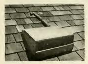
Take a couple of one by six-inch boards and cut them the same pitch as the heel of the rafter so that when they set on the roof they will make a level seat. Now take two wide shingles and nail the thick end of one on one of the one by sixes and the thin end on the other, and the other shingle nail it on just opposite, then brace the seat out on the end with two narrow shingles as shown in the picture.
