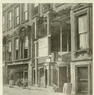
Fig. 4-Showing a Front Wall Shored and Needled at the Level of the Second Floor
