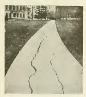
Such Work Is Inexcusable Here—Had the Walk Been Located on a Less Pretentious Spot, the Poor Workmanship Might Have Been Accounted For—On a State Campus Within Stone's Throw of Fine Buildings, This Walk Keenly Reflects Against the Institution
