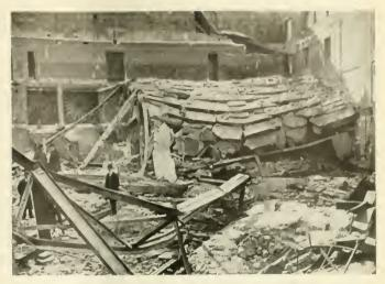
The Only Portion of the Reinforced Concrete Balcony to Partially Remain. One of the Roof Trusses Shown at Bottom of Picture; Note Ita Crumpled Condition.
