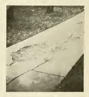
Here the Cracks Have Started the Walk to Crumbling, and, Aided by Frost, Has Wrought Havoc With What Should Have Been a Lasting Job—Imperfect Bonding of the Surface and the Body and Unclean Materials, or Possibly a Poor Grade of Cement, Might Account For the Damage
