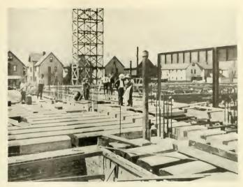
The Steel Pan Forms Placed in Position on the Channels, When All Are Set the Job Is
