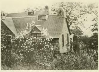
This Roof Is Just Plain Rubberoid Roofing, Laid in Horizontal Strips-The Shingle Effect
