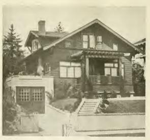
An example of making the most of the site. The problem of the house and garage on a small lot has been carefully handled here. The roof of garage forms a terrace for the first floor rooms.
