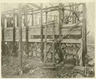
The Forms Used for Laying Up Masoury Walls-All Parts Are to Be Used as Permanent Construction Equipment-They Also Serve as Scaffolding
