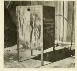
Several modern heating devices have been made available recently. This heater, in addition to its function as a salamander for kerping the enclosure warm where desired, contains a coil of pipe by means of which the water may be heated to a desired temperature
