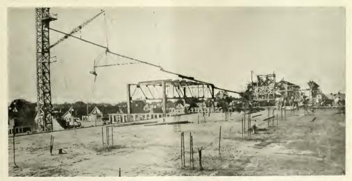
Chuting the Concrete For the Beams and Floor-Notice the Elevator Tower With a Substantial Ladder On Its Side-Safety First
