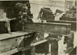
Fig. 6-Basement Wall Needled with Beams Set in Pairs, Steel Beams for Support of New Wall
