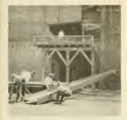
Heavy Steel Beam Being Moved in Position to Hoist in Outside Elevator Shalt
