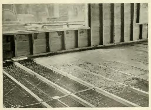
How the Concrete Floor Is Laid on Mctal Lath. Note the Sleepers for Nailing Wood Floor
